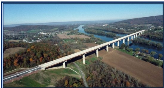
The Central Susquehanna Valley Transportation River Bridge in Northumberland County Photo by PennDOT Photogrammetry and Surveys Section
