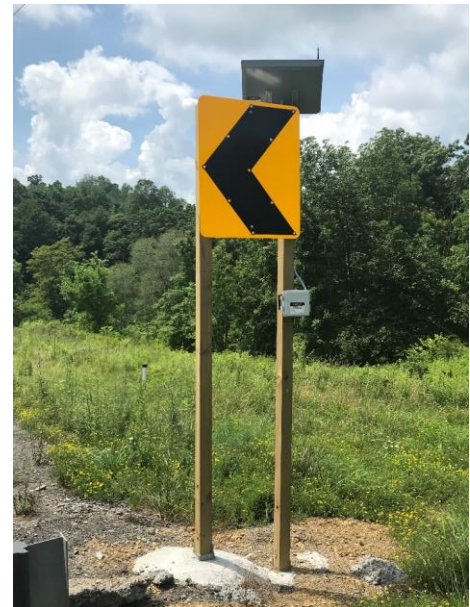
All of District 11’s ground installations currently utilize wooden poles set in concrete as shown. In the future, staff will consider metal cast bases instead to simplify replacement.
