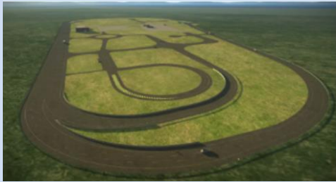
PennSTART is a state-of-the-art training and testing facility for the Mid-Atlantic region.
