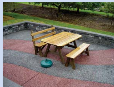
Pervious Pavement is approved for use in parking lots, sidewalks and trails.
