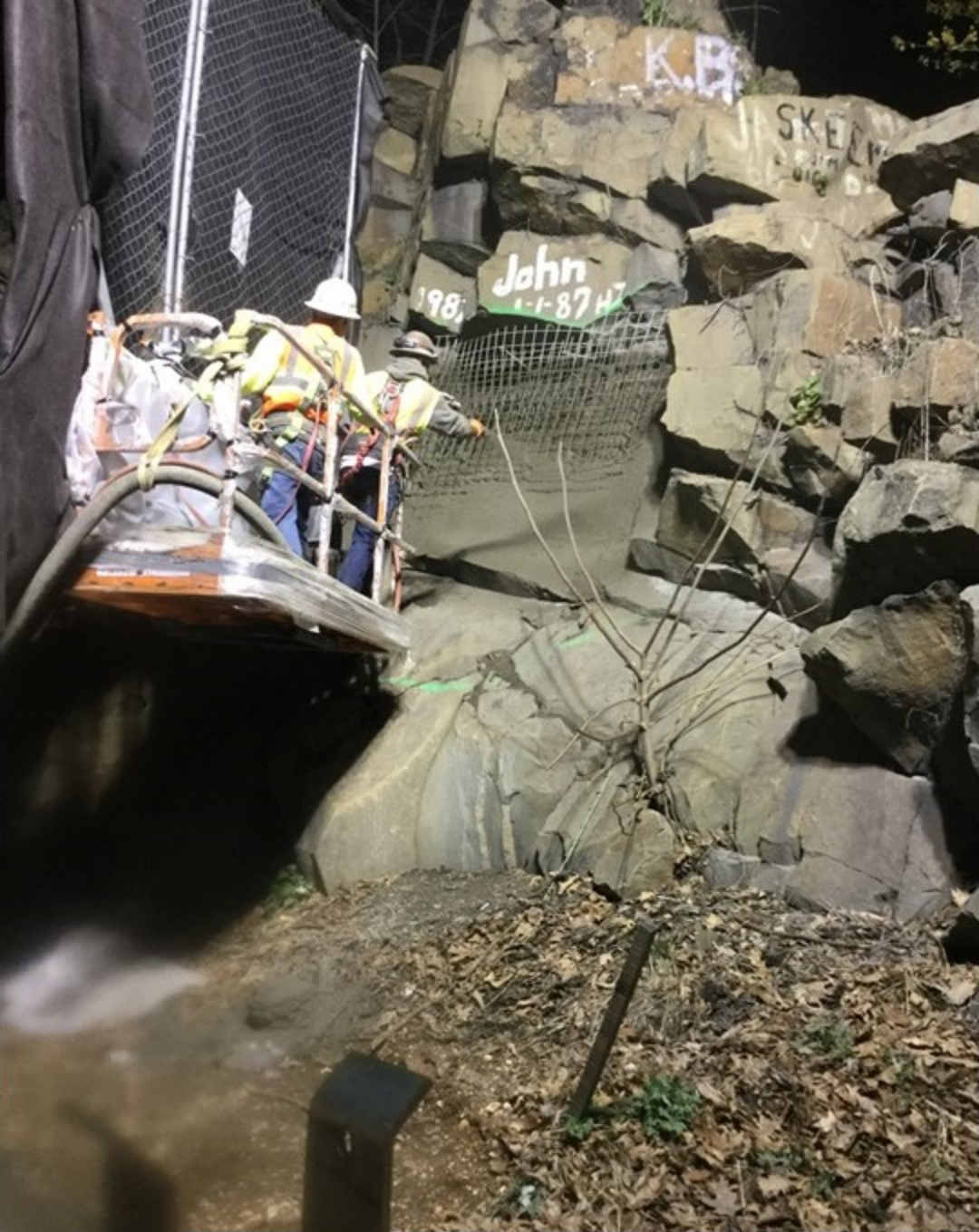
Shotcrete application for rock overhang supports
