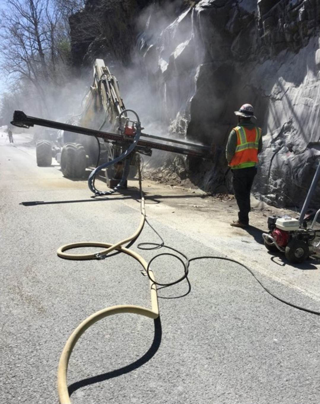
Pre-Closure anchor bolt drilling
