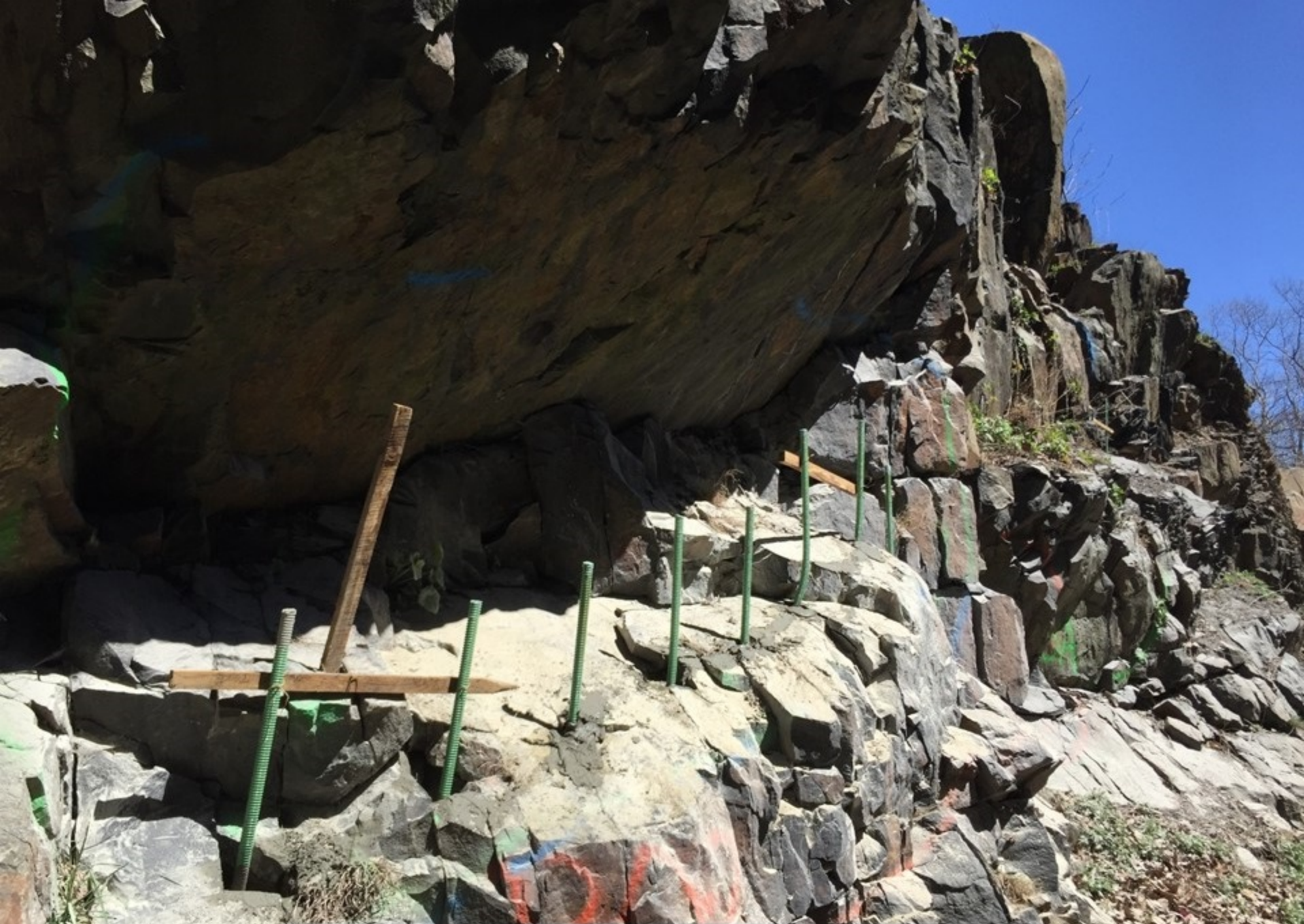
Rock overhang support dowel installation
