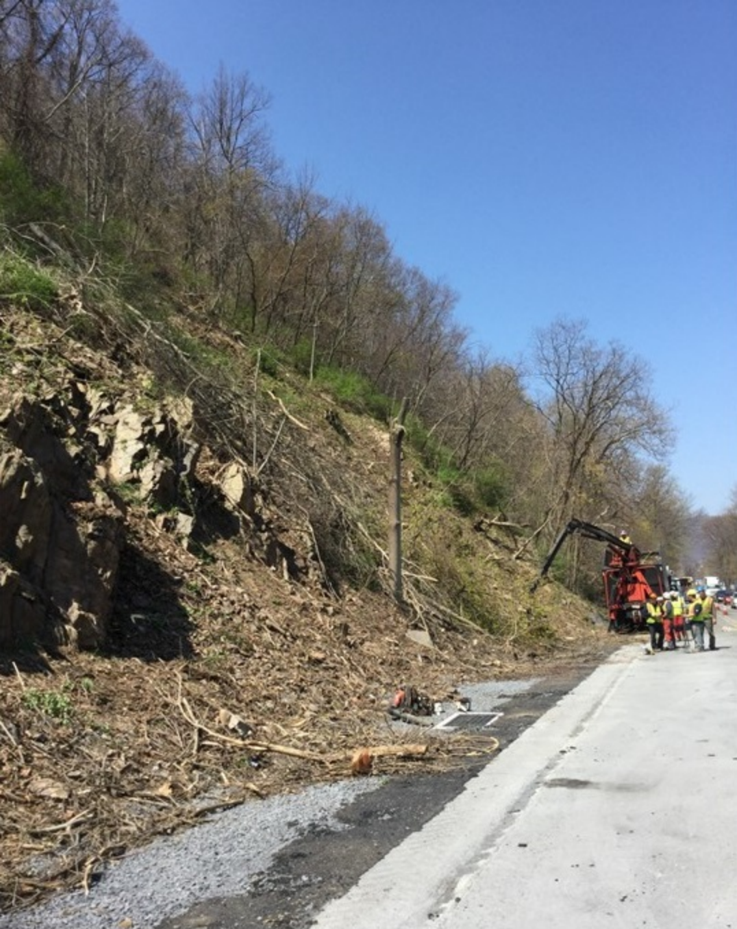
Pre-Closure tree clearing
