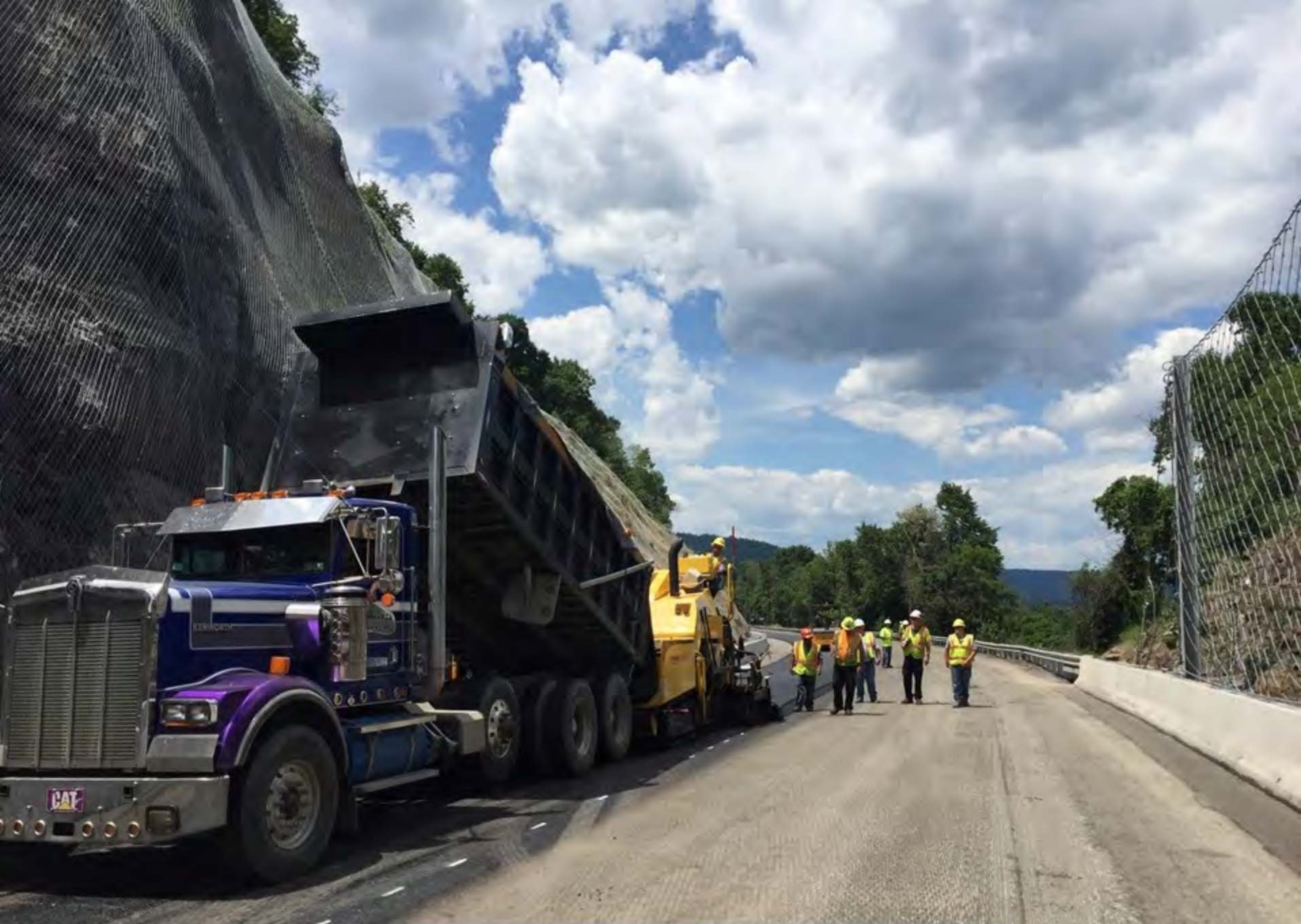
Bituminous paving at southern cut
