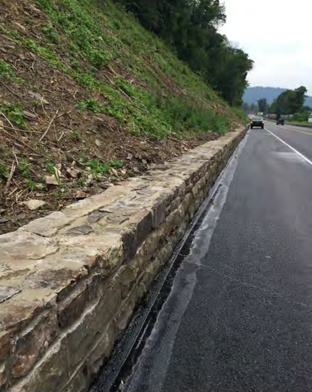
Restoration work completed on existing stone wall
