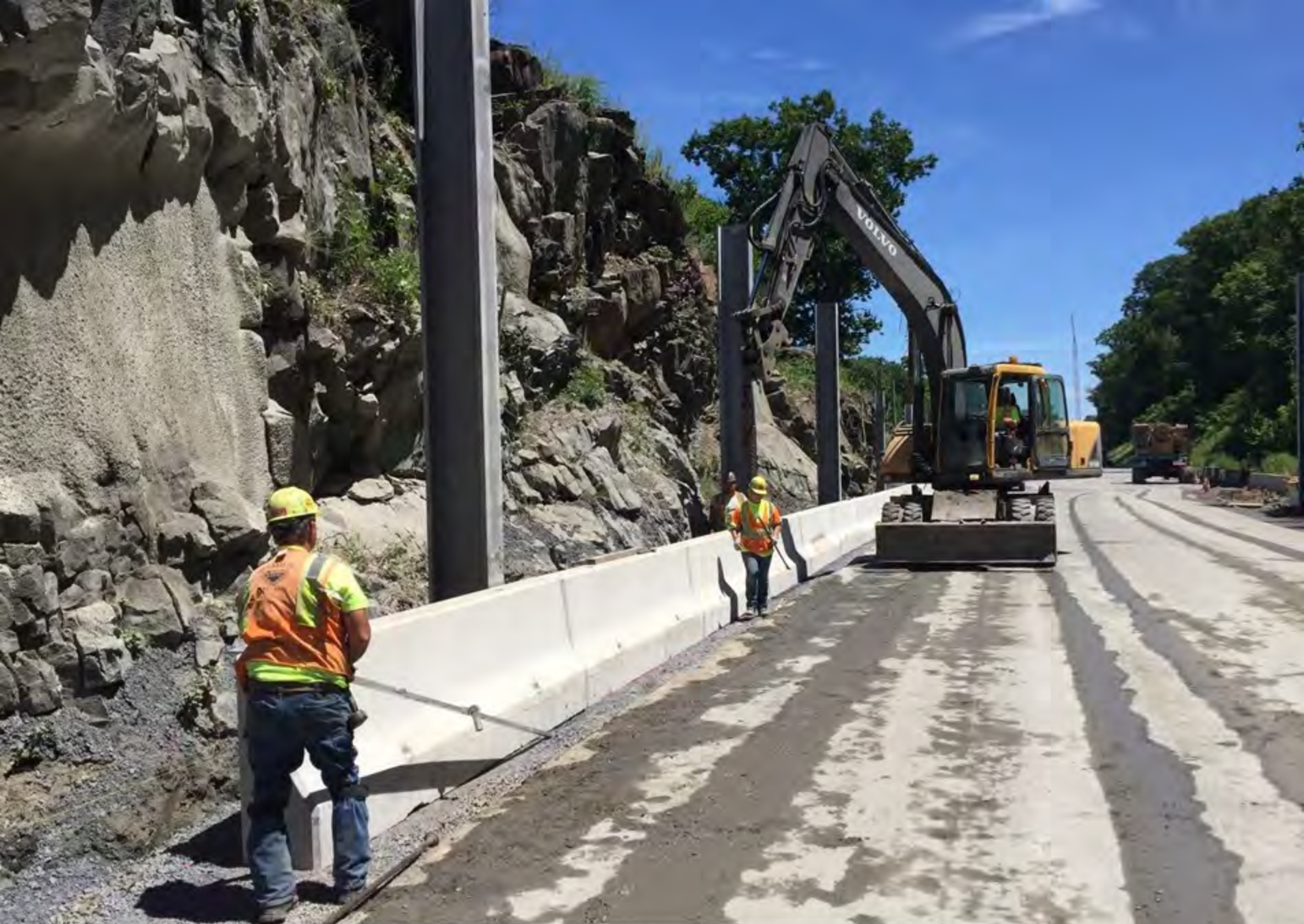
Concrete barrier placement
