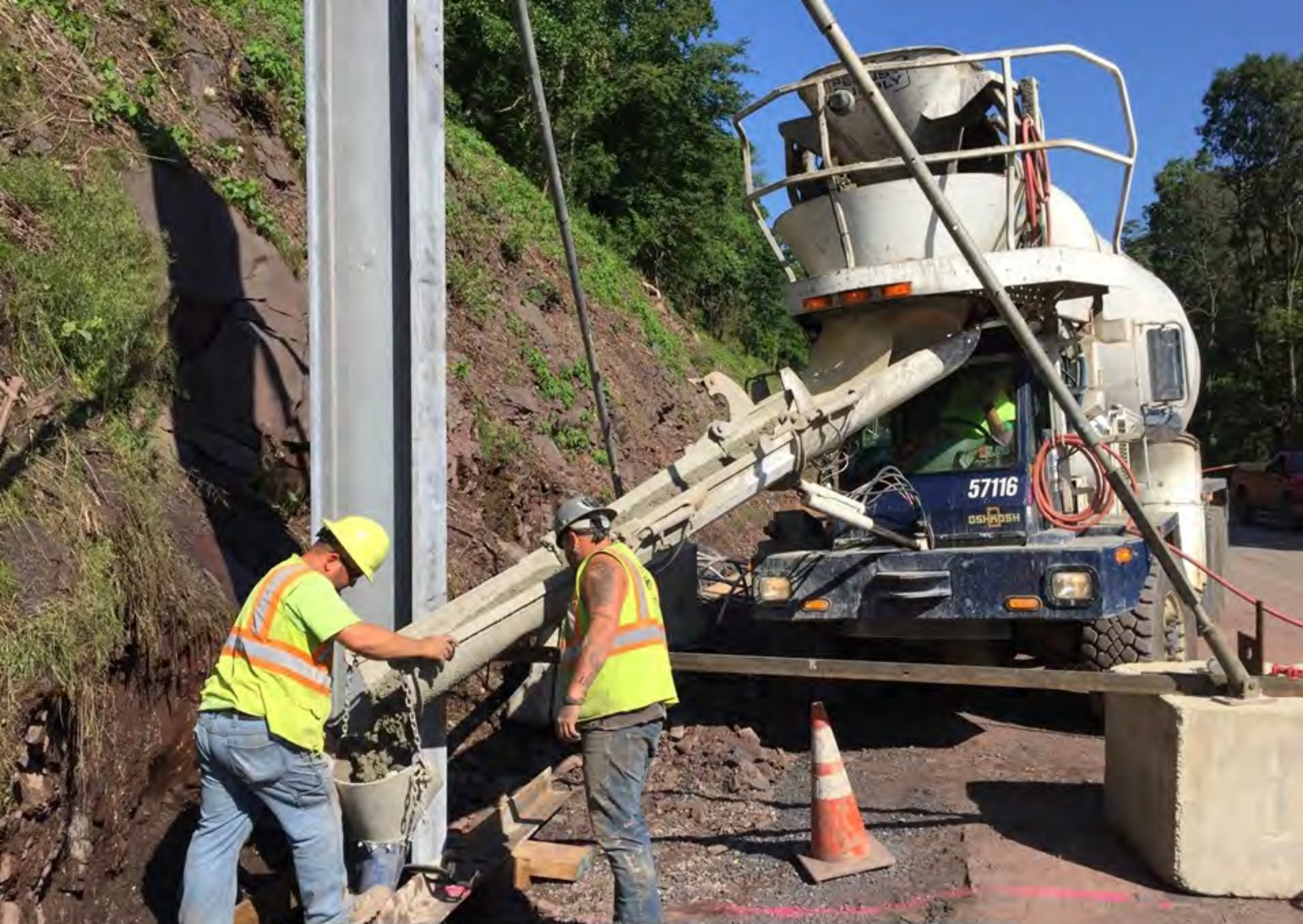
Rockfall fence post caisson concrete placement
