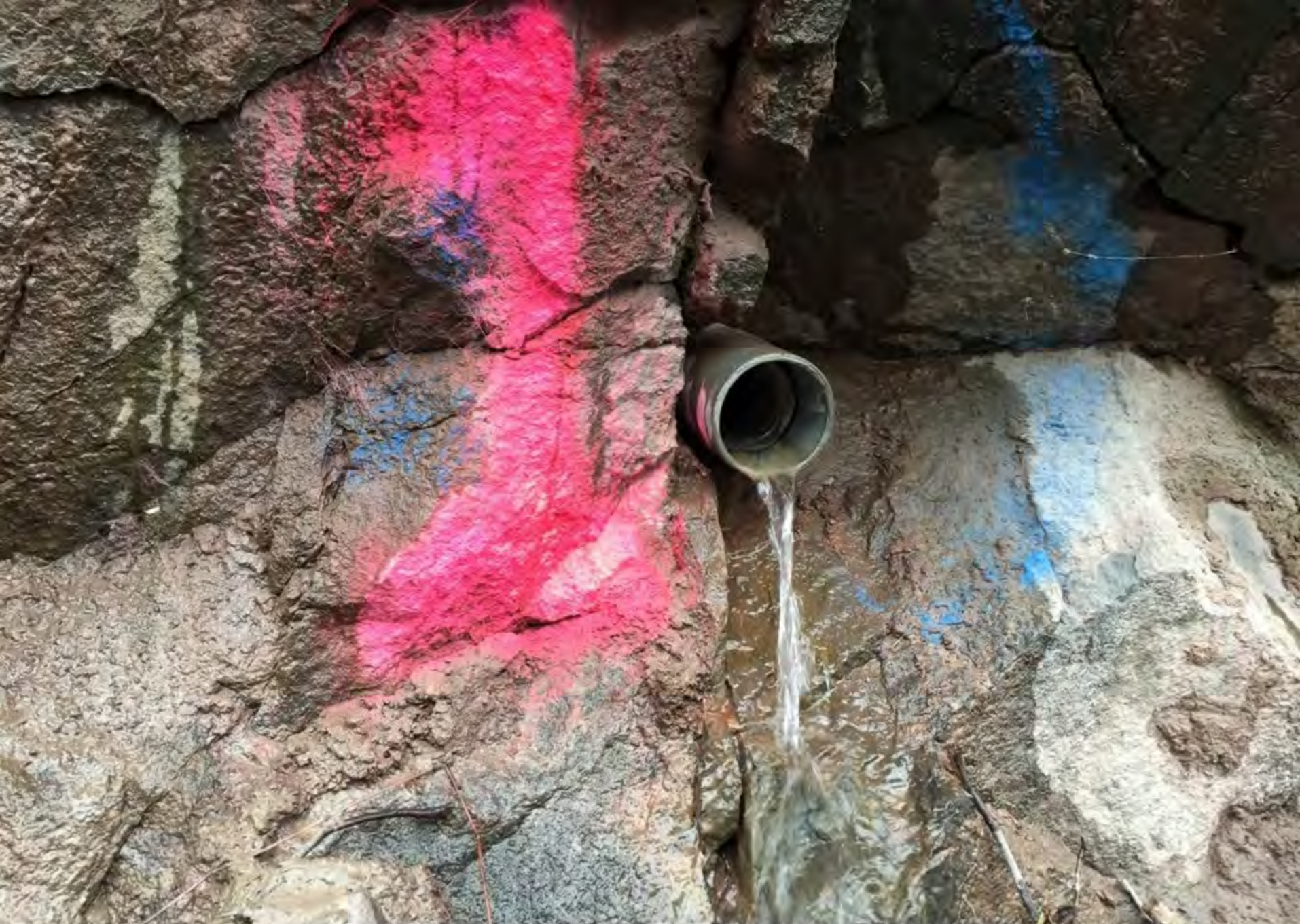
Perforated pipe installed to drain water from slope
