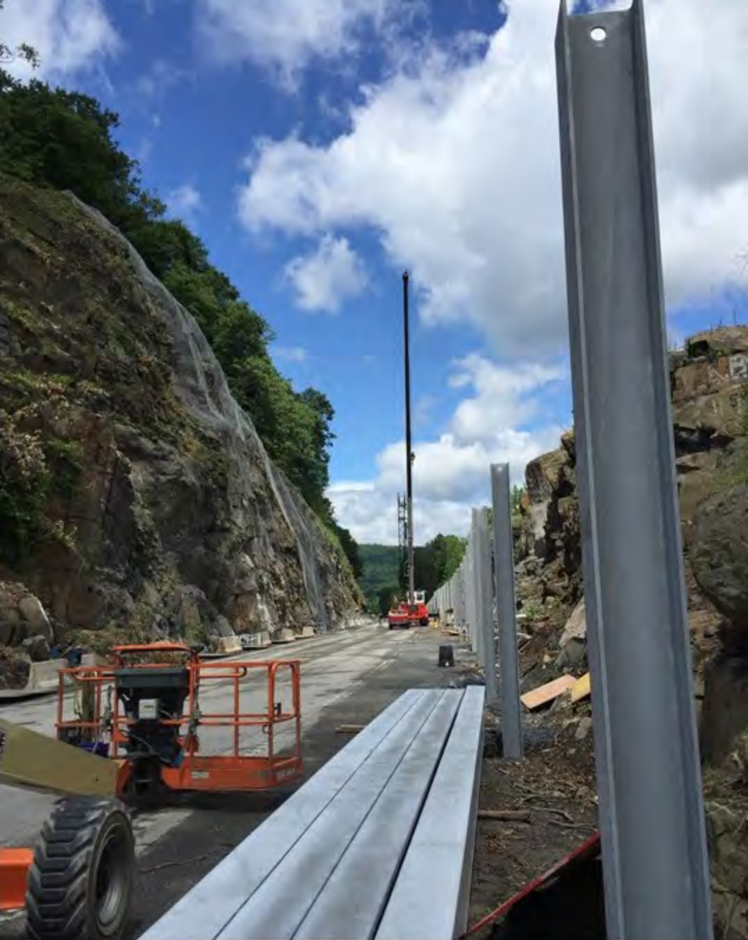
Rockfall fence posts at northern cut
