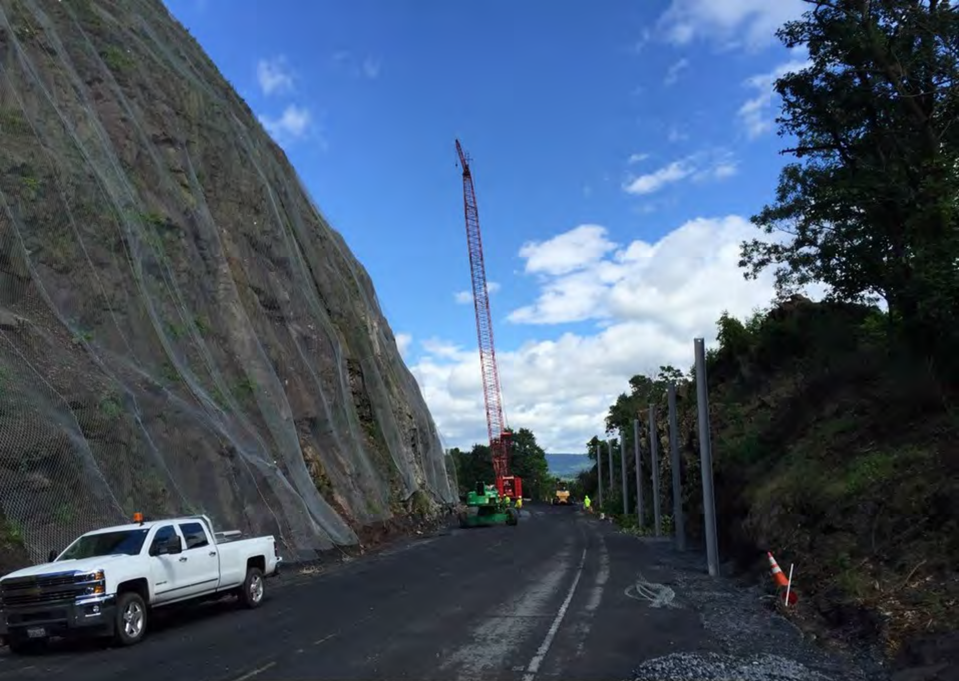
Mesh installation at southern cut
