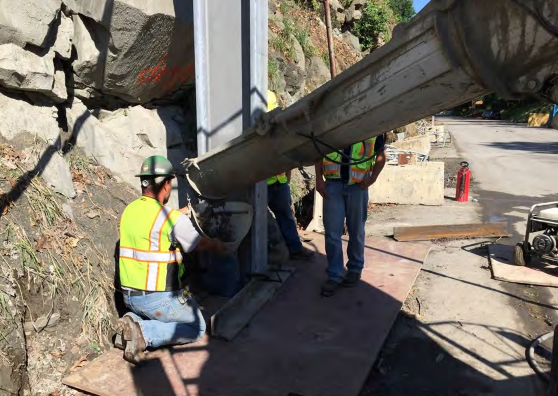
Rockfall fence post caisson concrete placement
