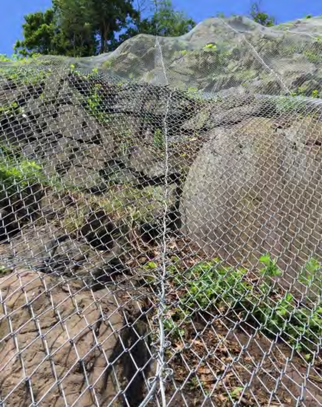
Steel cable lacing of wire mesh
