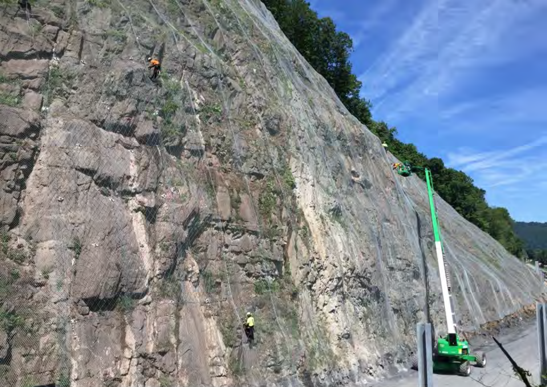
Lacing mesh at southern cut
