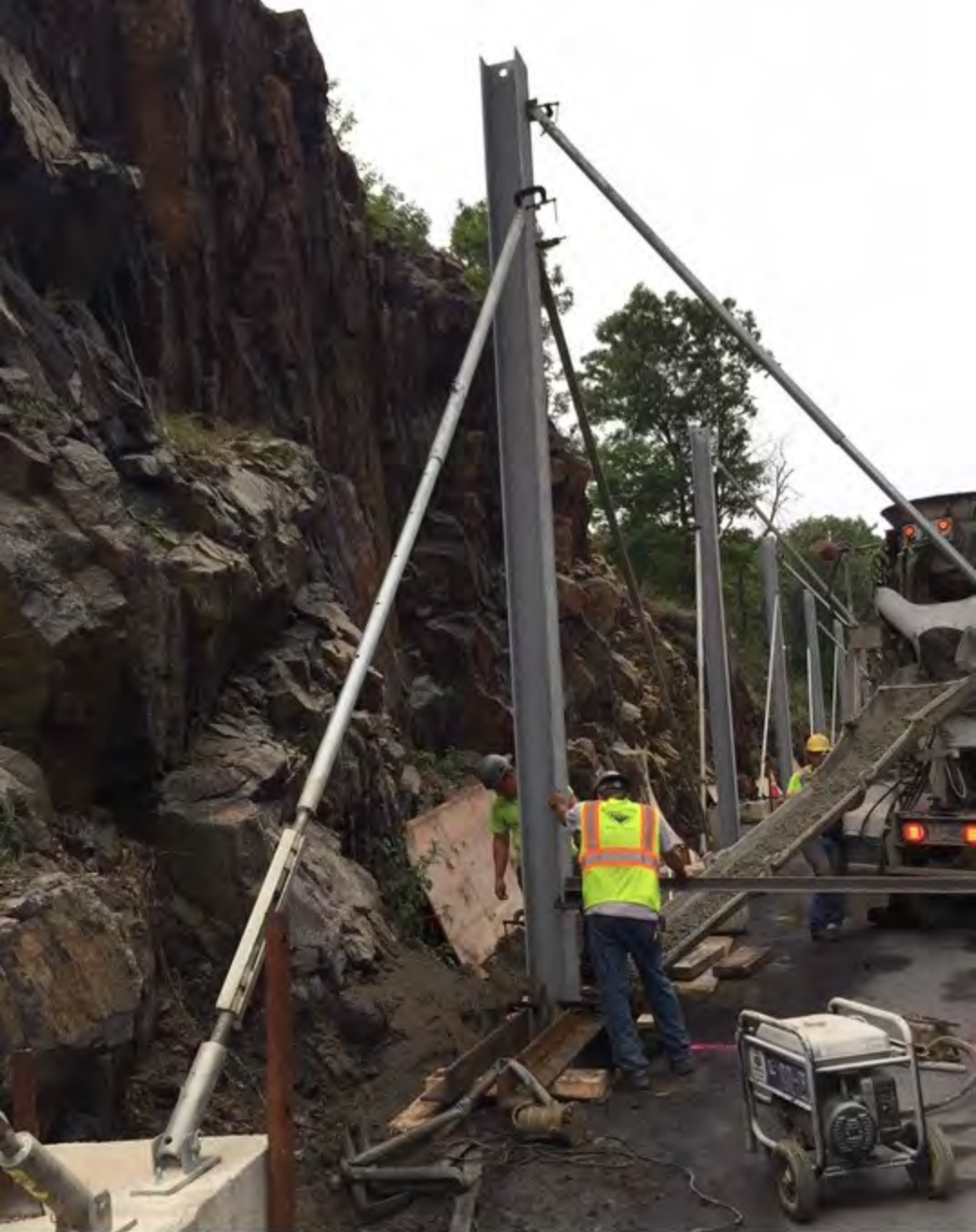
Rockfall fence post installation
