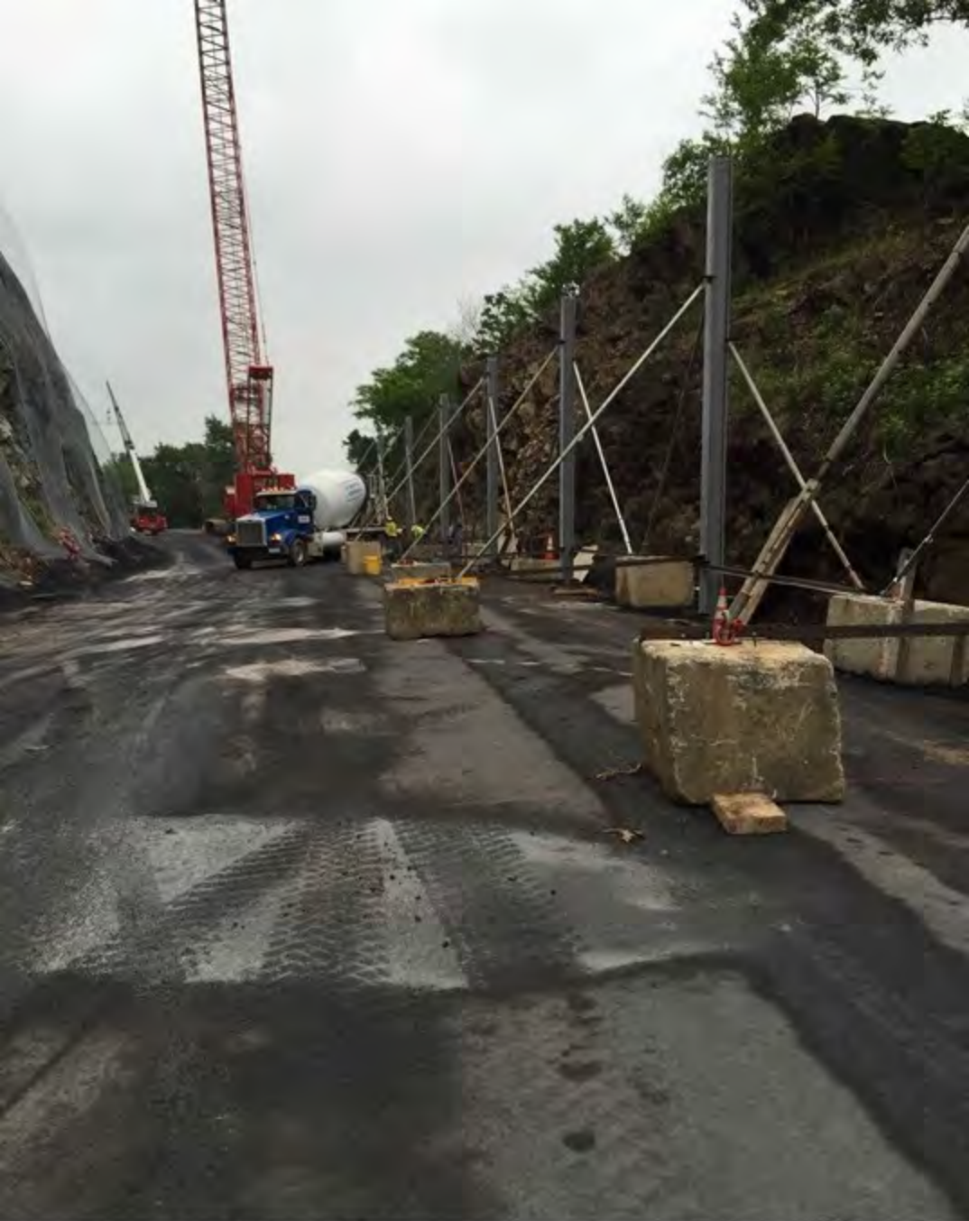
Rockfall fence post installation
