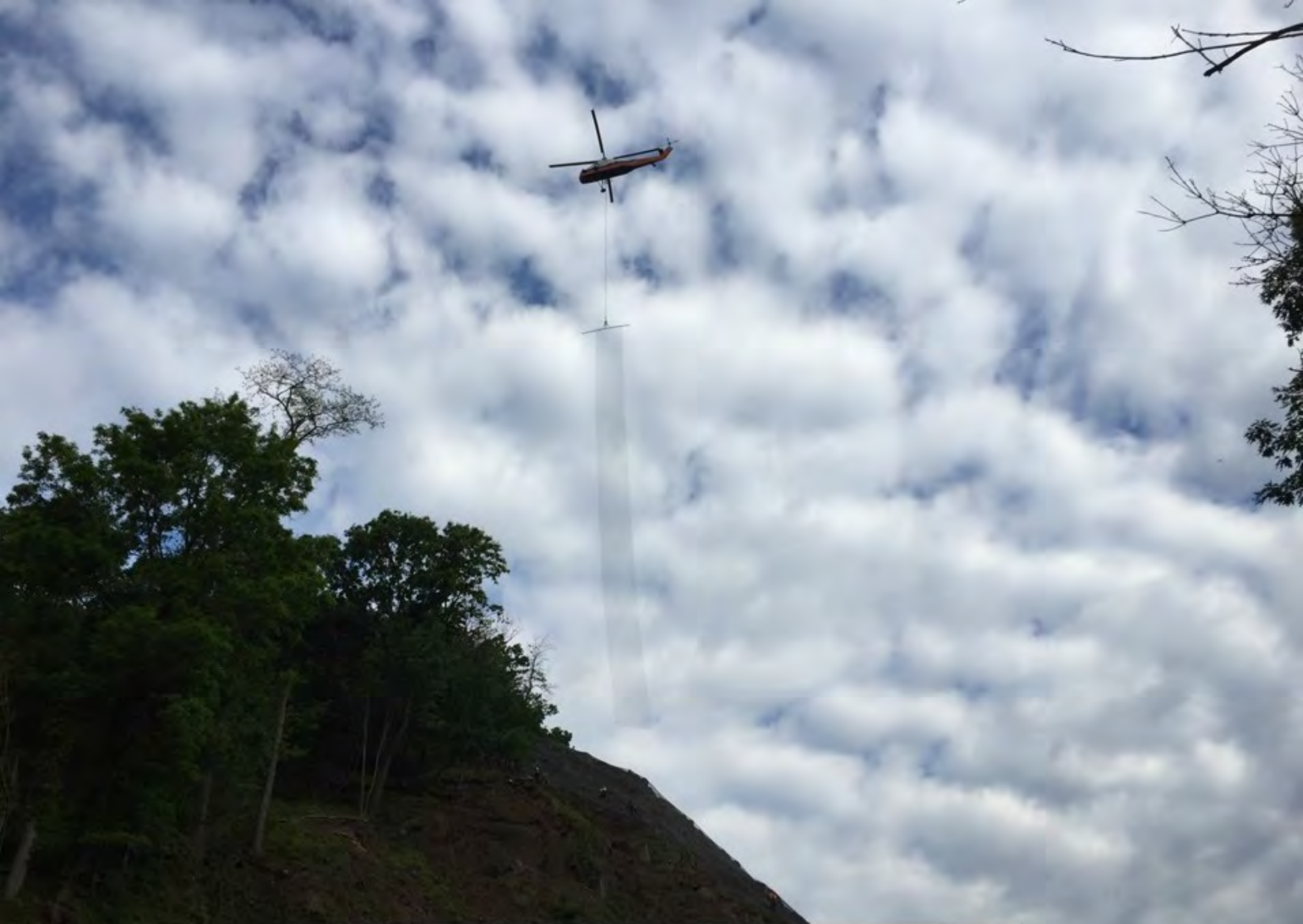
Helicopter placement of wire mesh on slope
