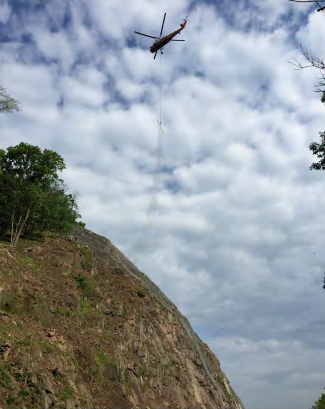
Helicopter placement of wire mesh on slope
