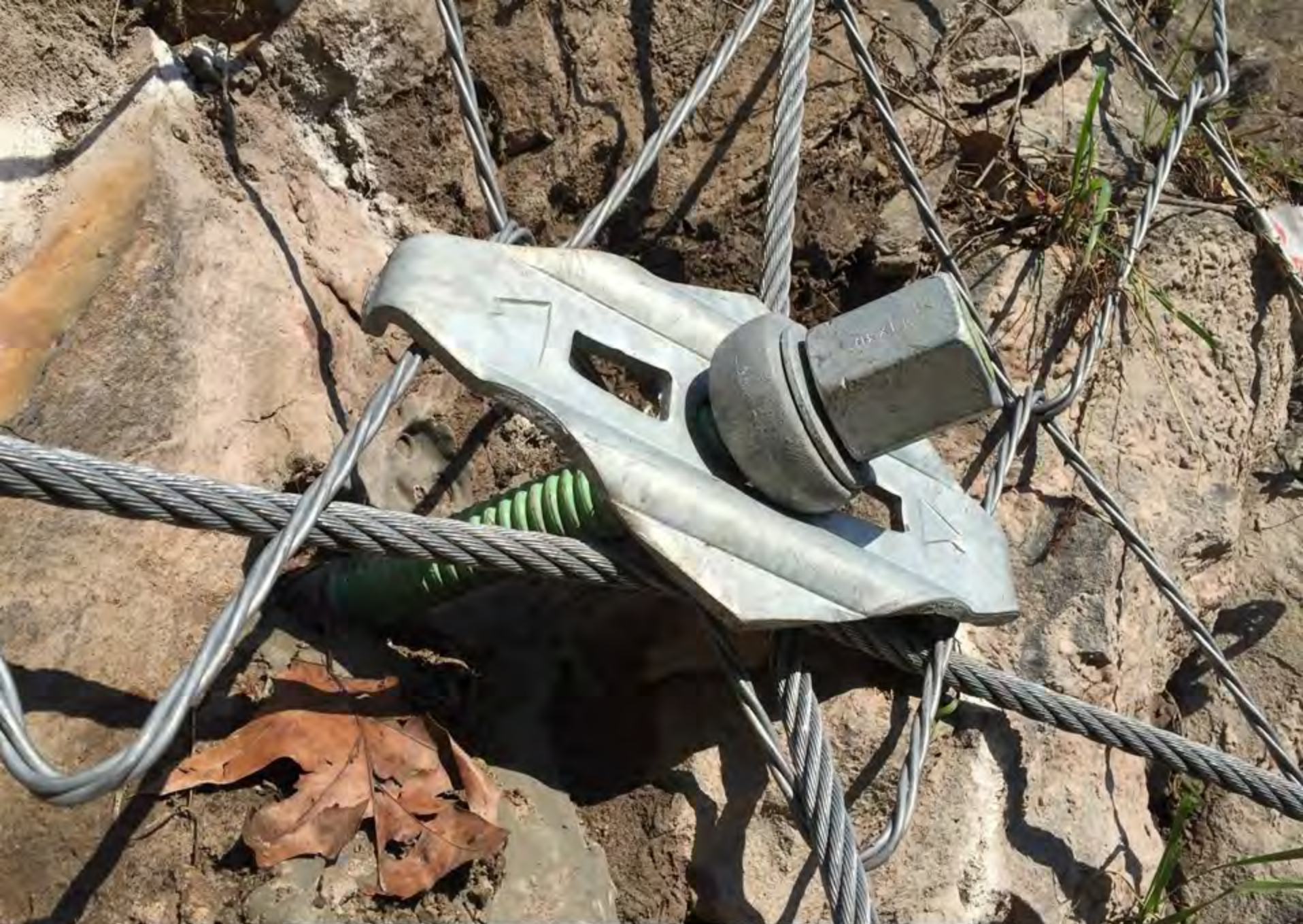
Spider Wire/anchor bolt attachment
