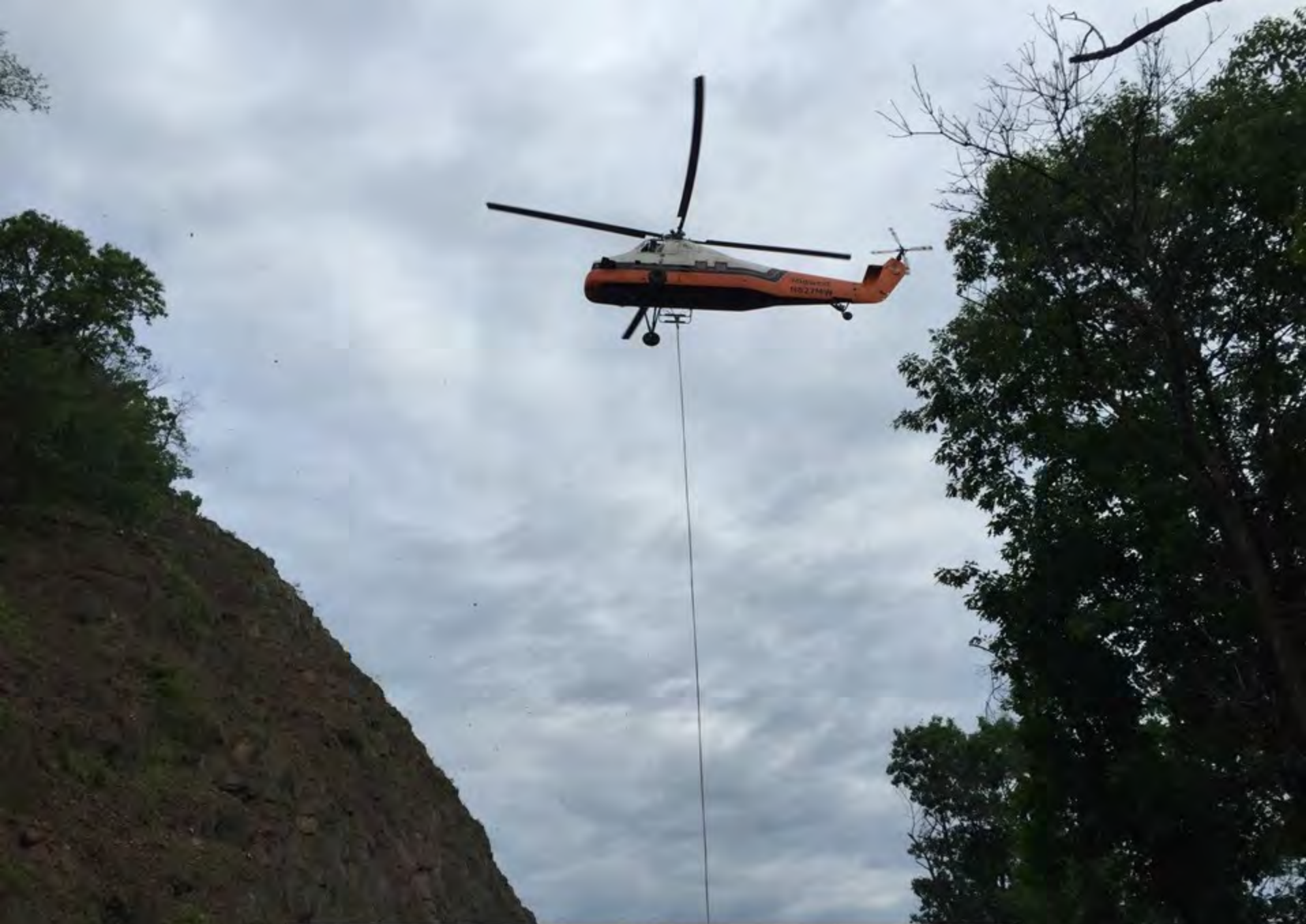
Helicopter placement of wire mesh on slope
