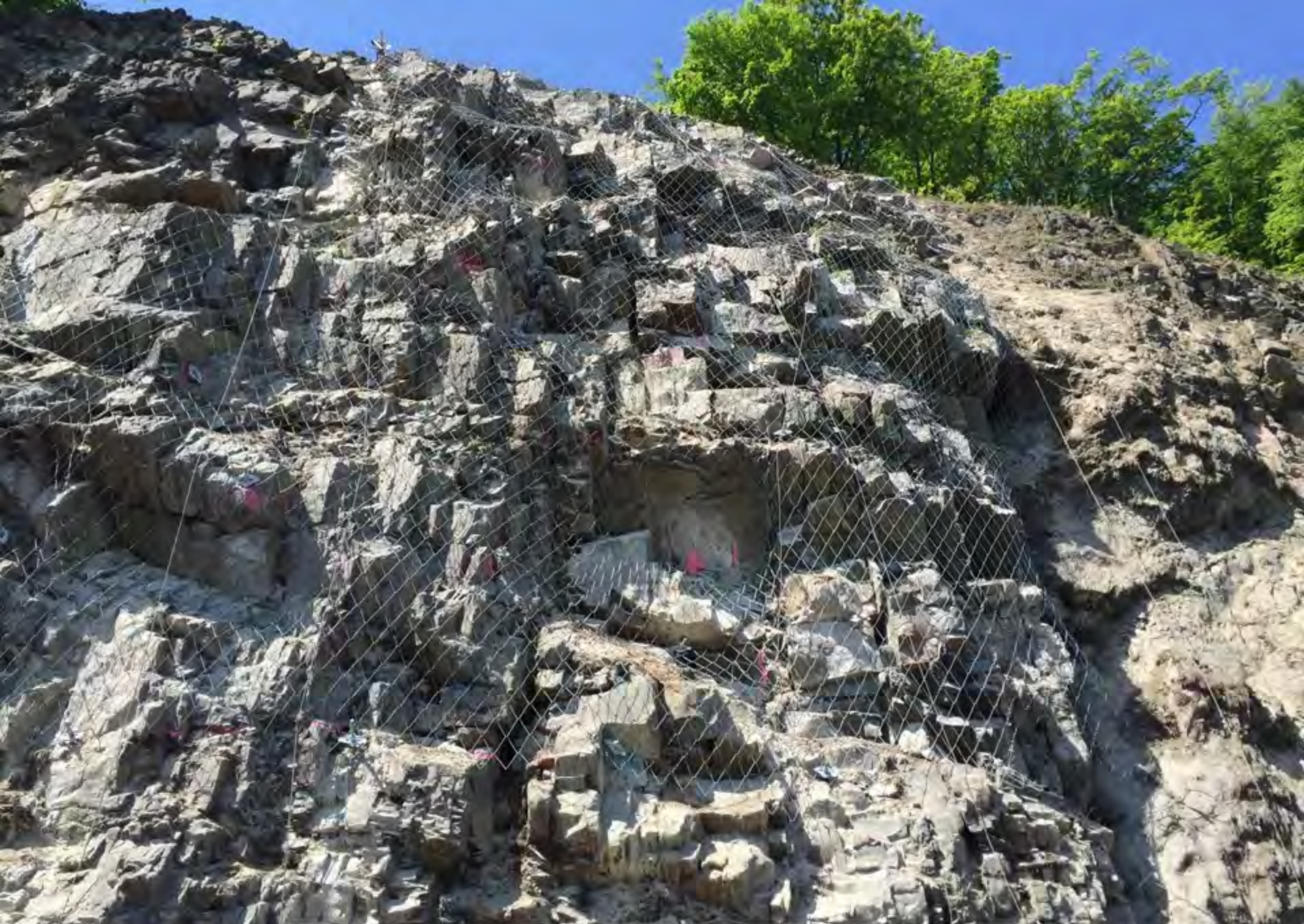
Spider Wire mesh installation
