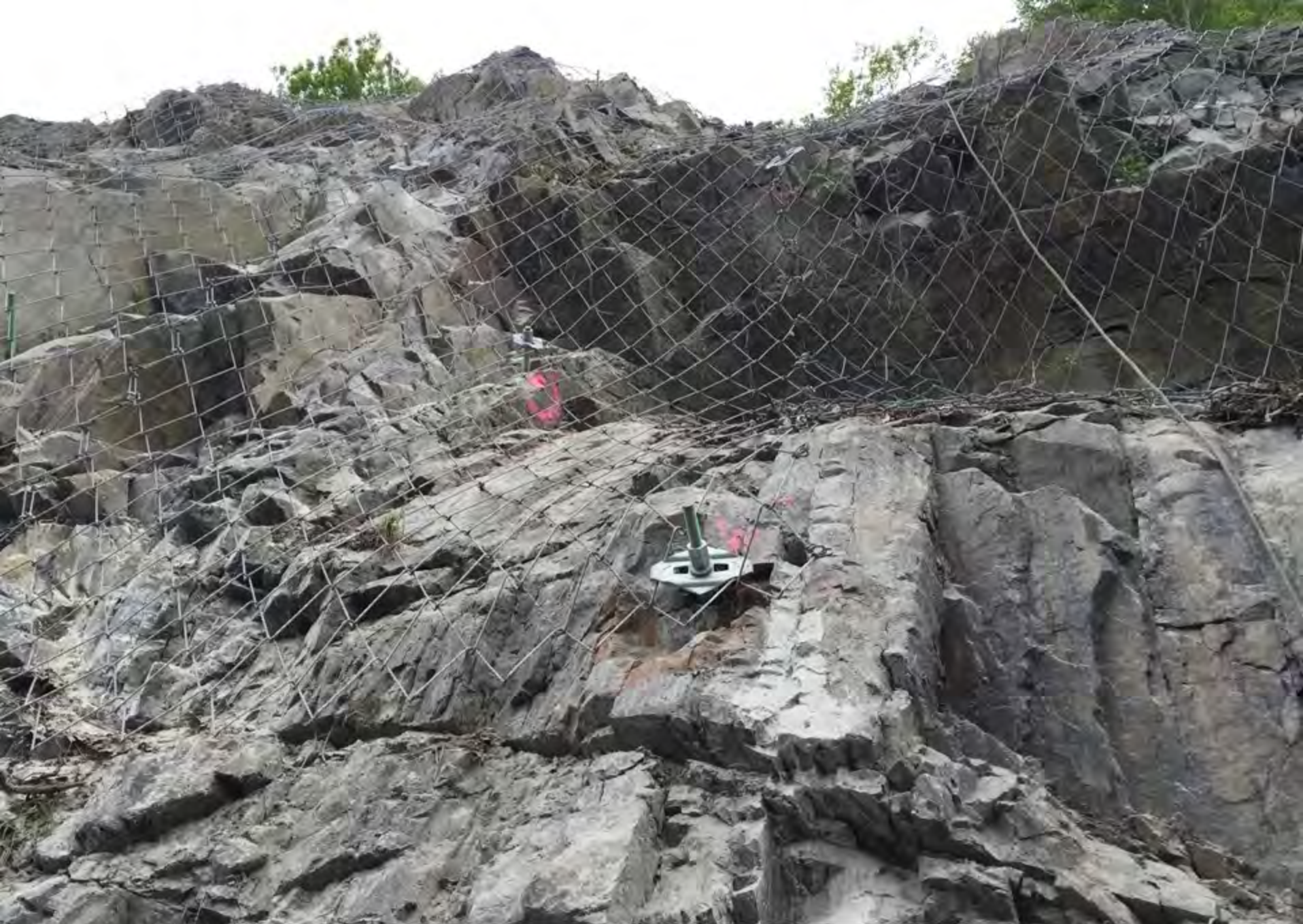
Spider Wire mesh installation at northern cut
