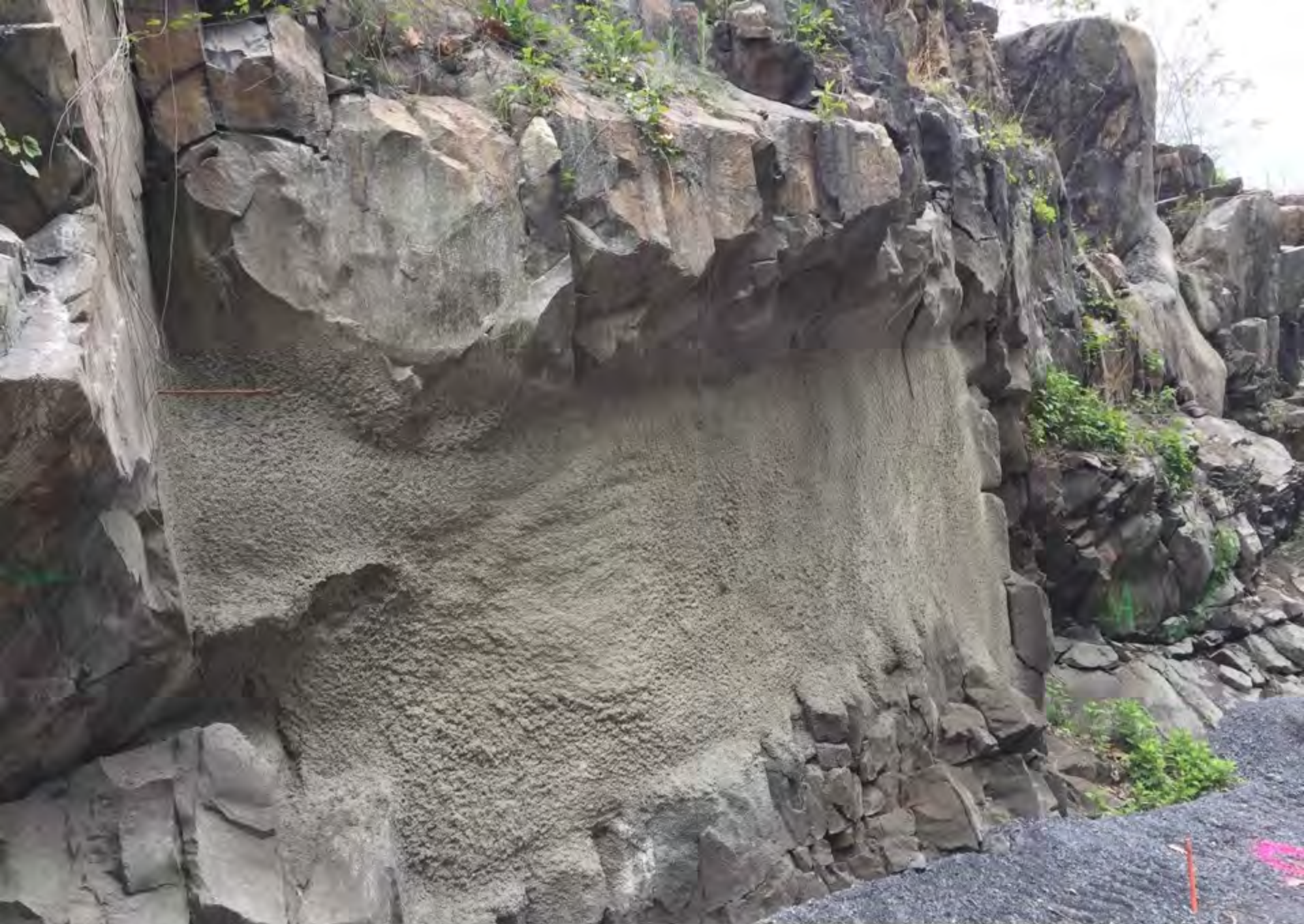
Shotcrete rock overhang support – to buttress void in rock
