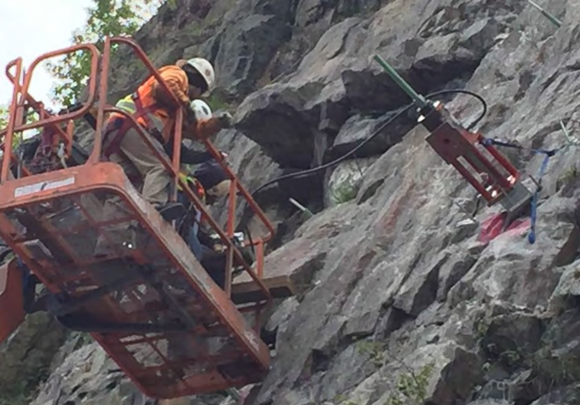
Performing pull test on rock anchor
