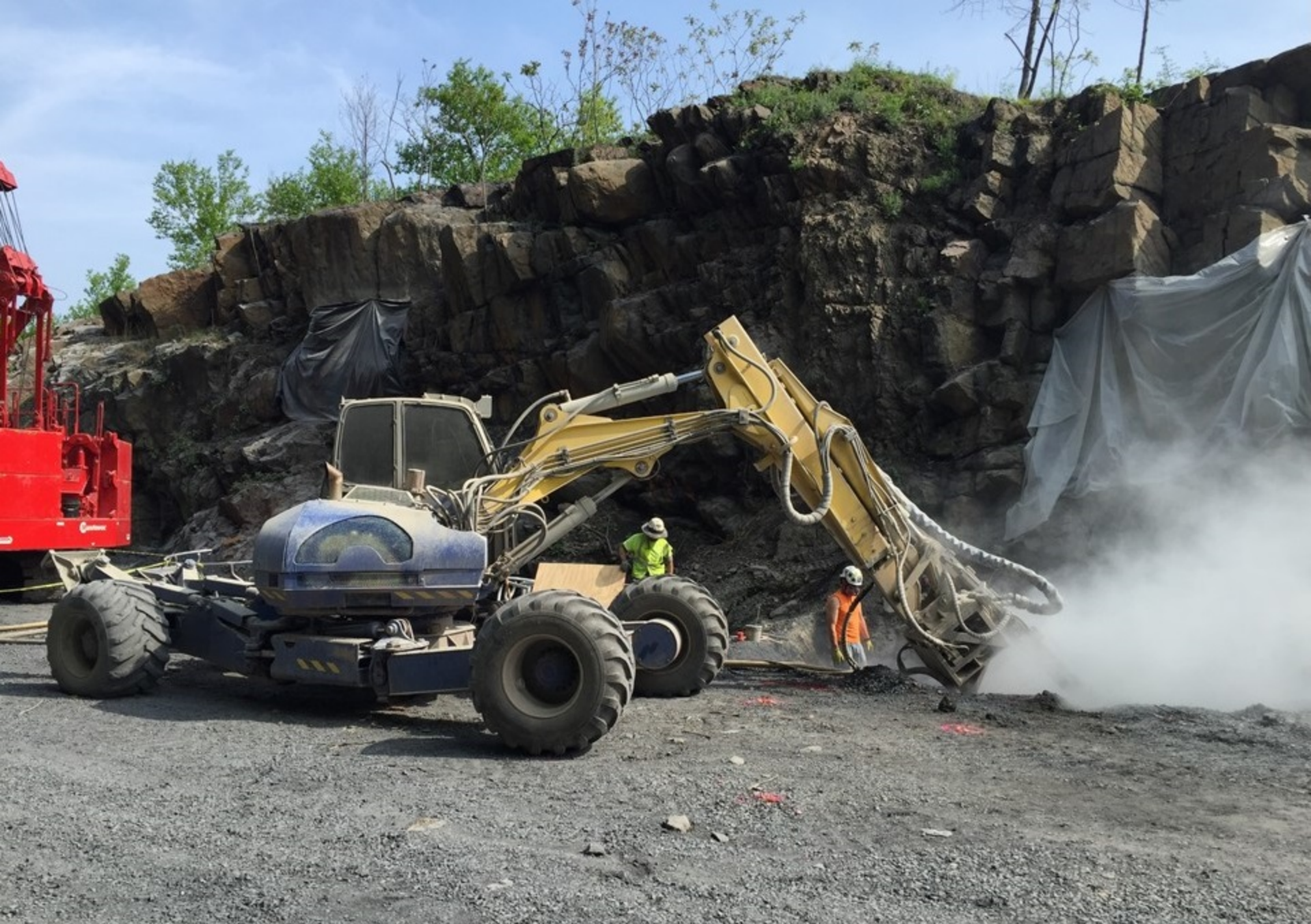
Drilling tie-backs for rockfall fence
