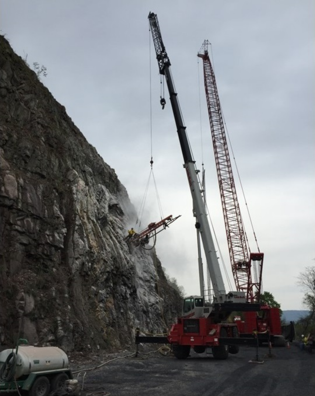
Drilling rock anchors
