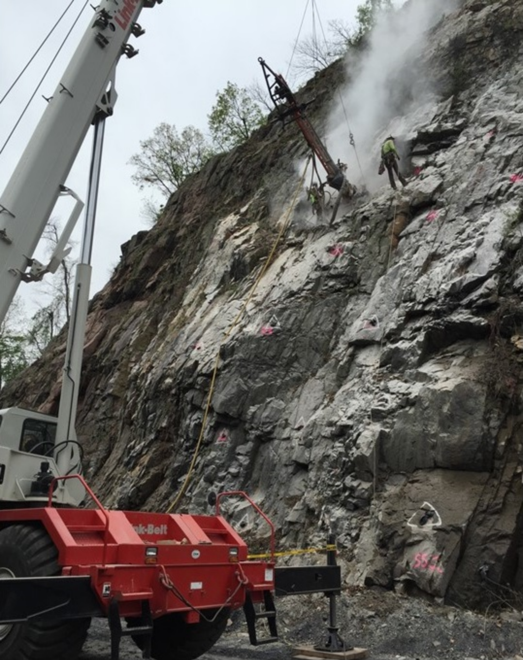
Drilling rock anchors
