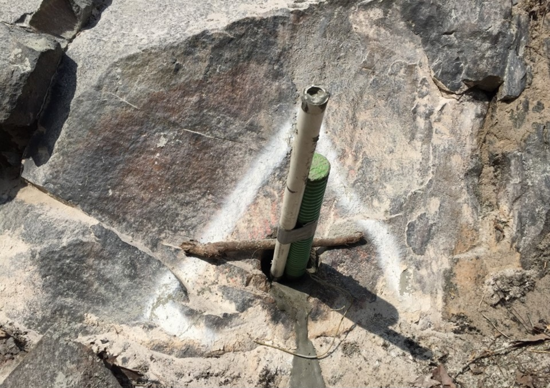
Grouted rock anchors
