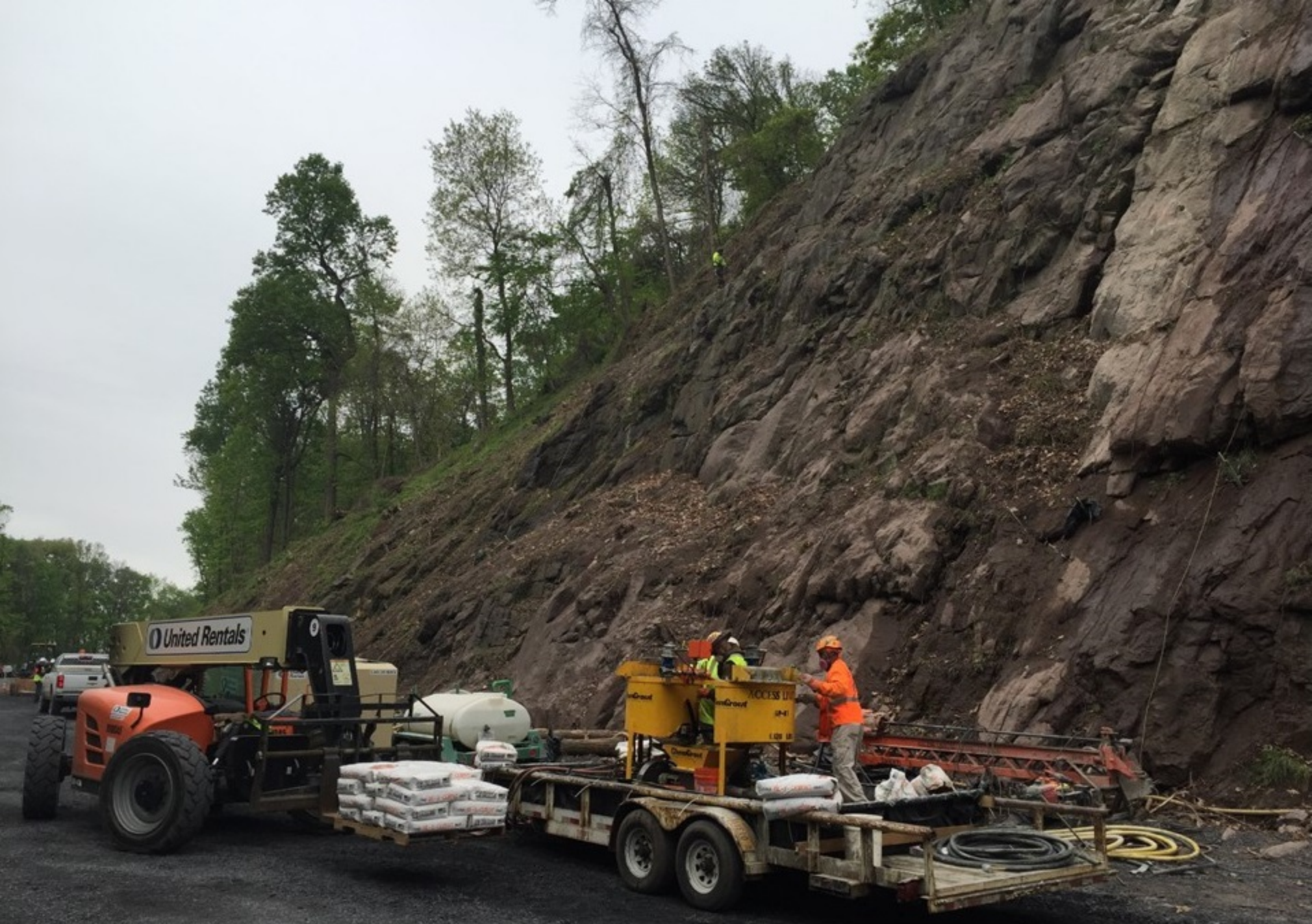
Grouting rock anchors
