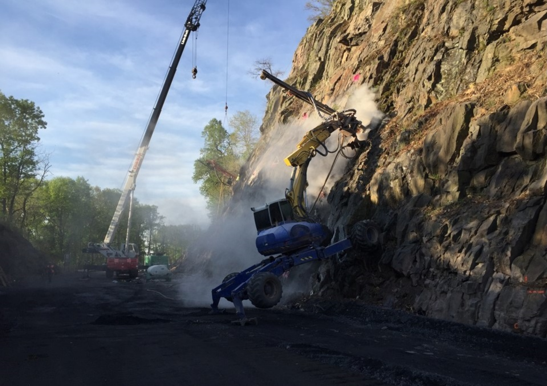
Rock anchor drilling at southern cut
