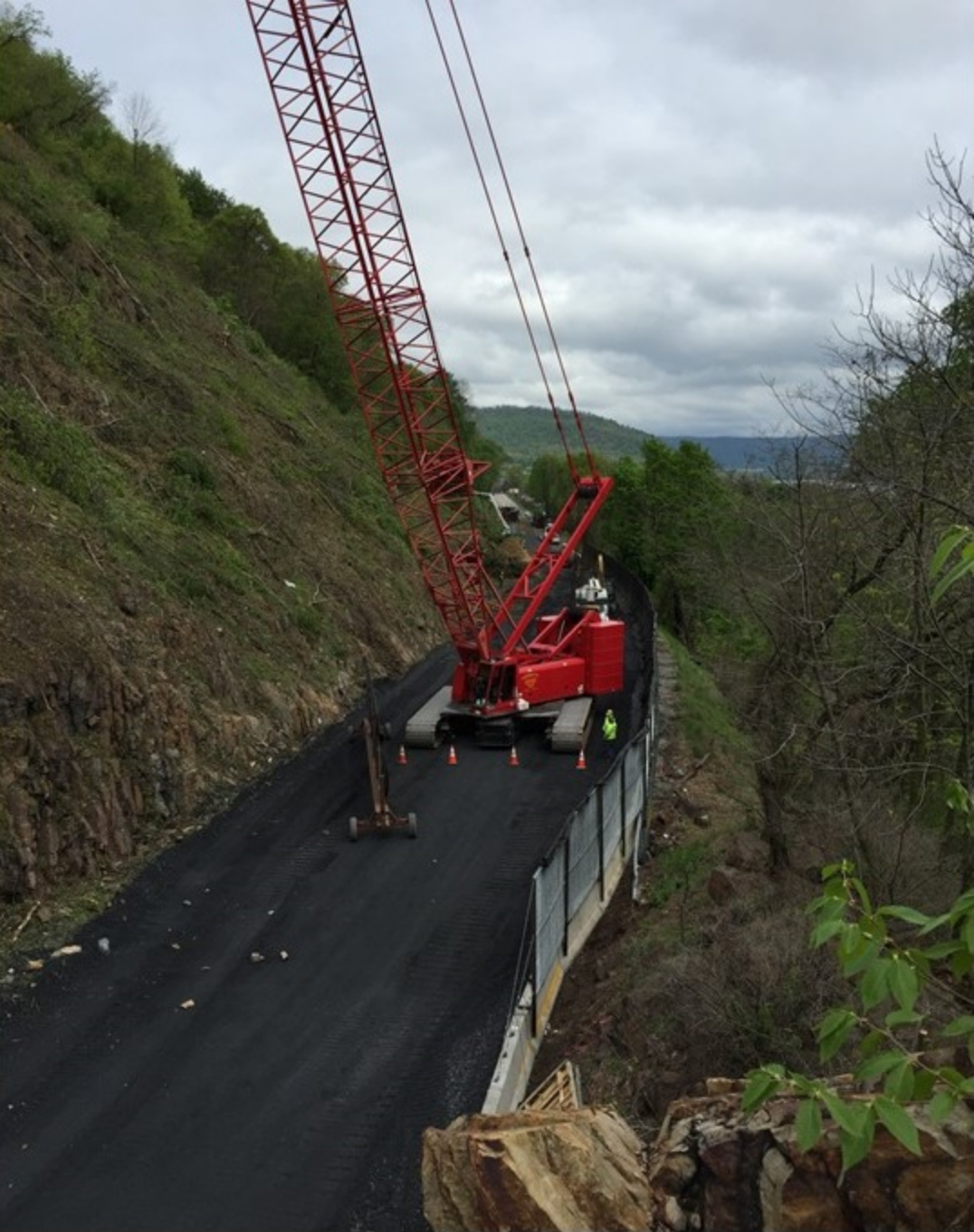
275 Ton crane and stone pad
