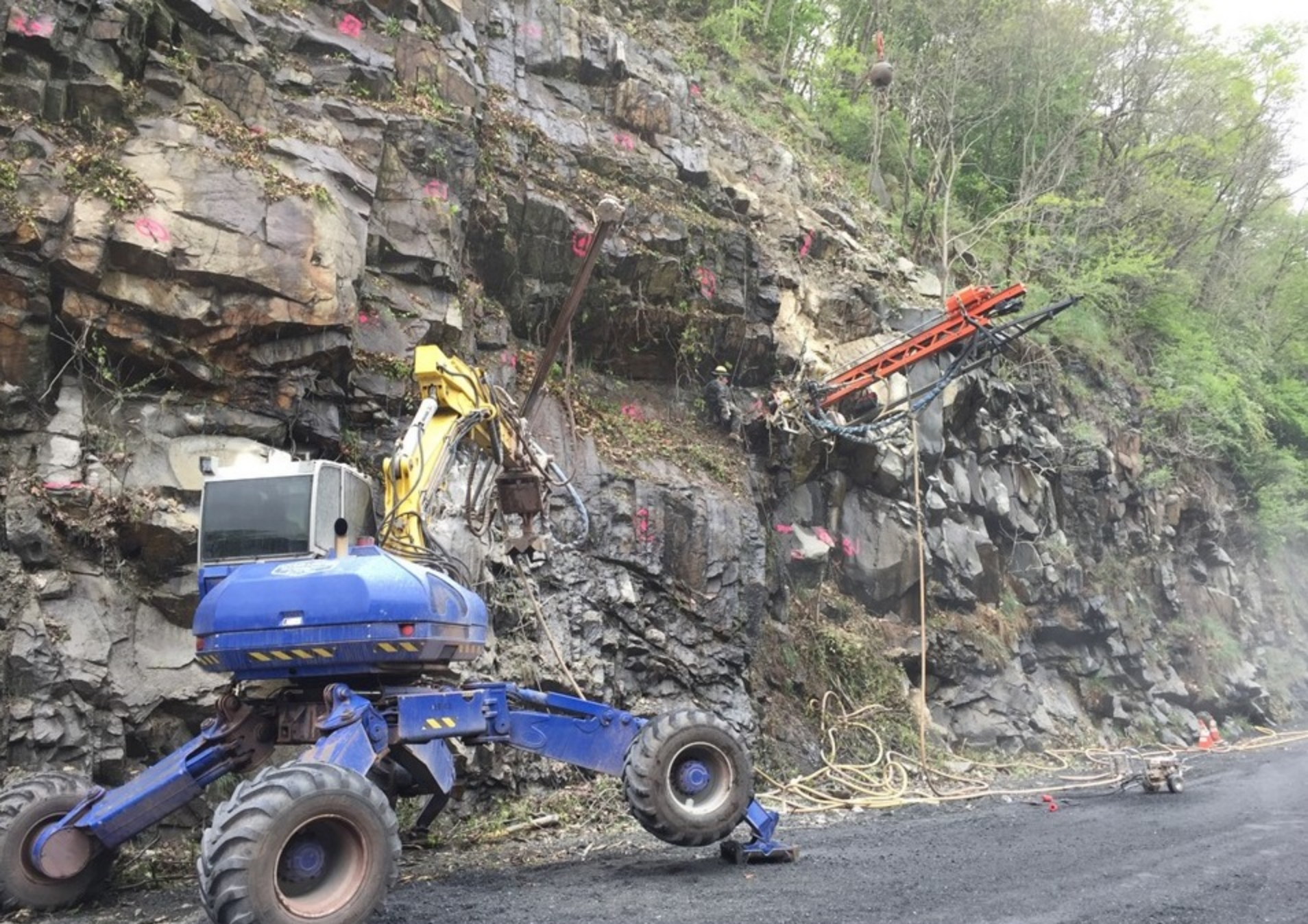
Rock anchor drilling at north cut
