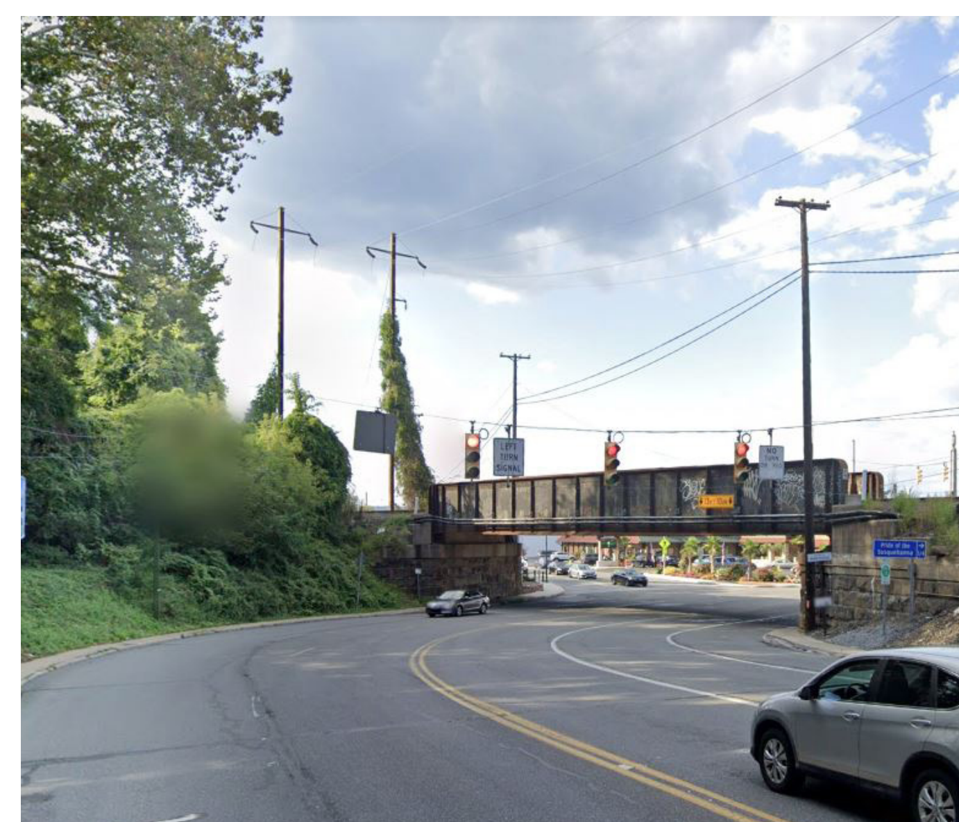
Approaching Front Street intersection looking eastbound
