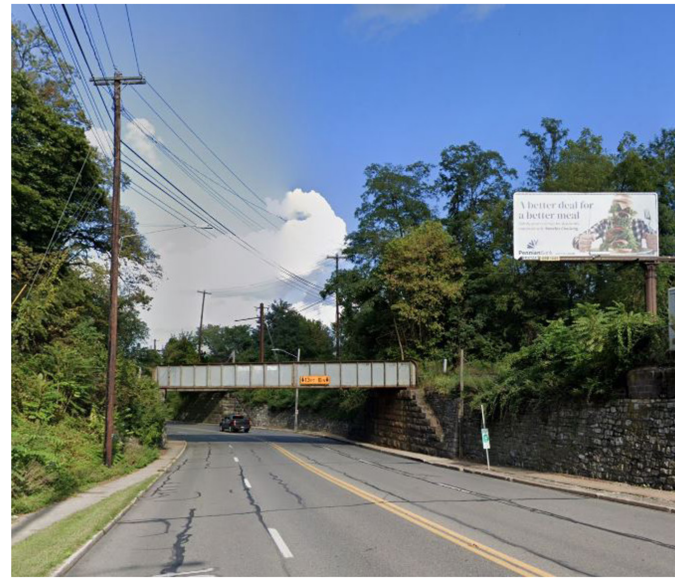
Approaching the main curve in the road looking eastbound
