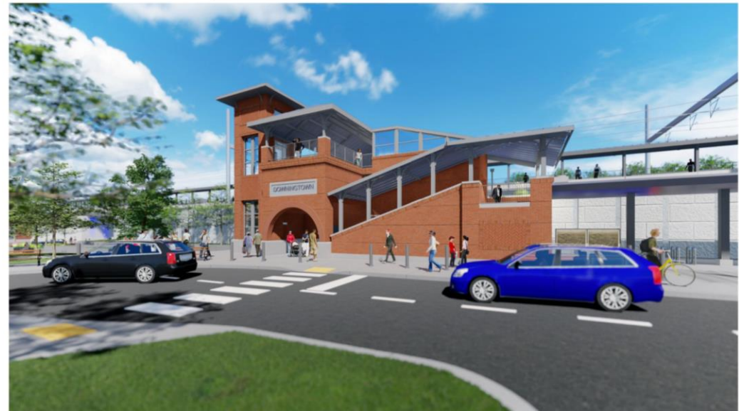
STATION - SOUTHEAST QUADRANT
