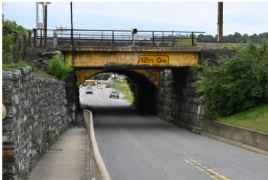
EXISTING BRIDGE - LOOKING SOUTH
