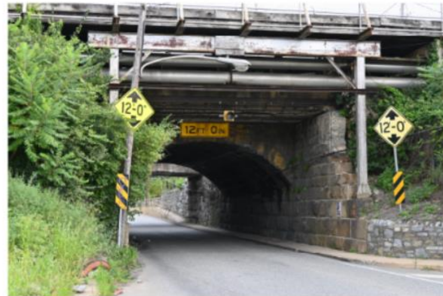
EXISTING BRIDGE - LOOKING NORTH
