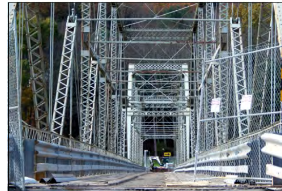
Struts and trusses.
