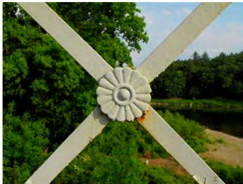
Flower motifs on bridge railings.
