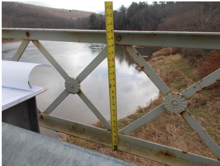
Photo 36 - Skidders Falls Bridge: Typical View of Decorative Railing
