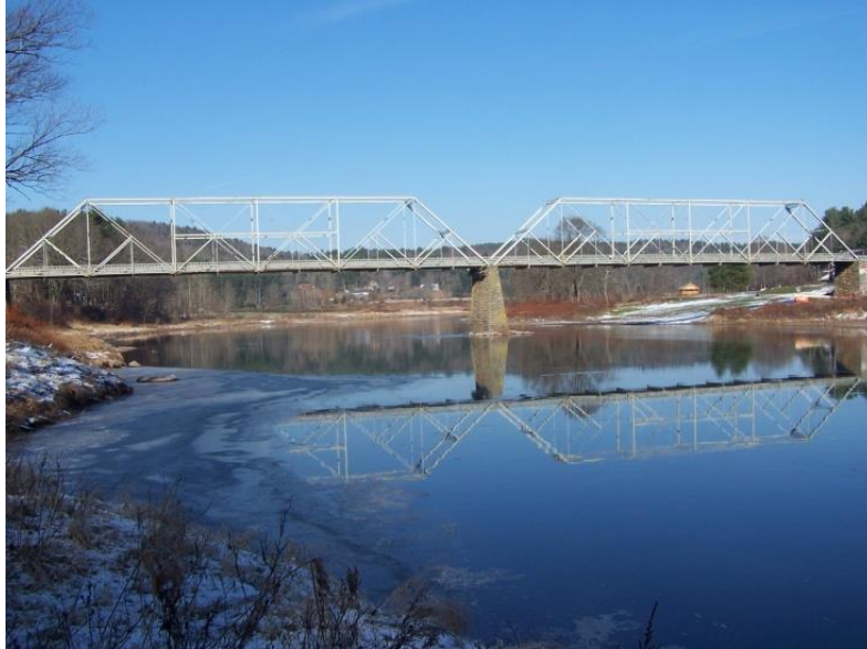
Photo 1 - Skinnners Falls Bridge: Downstream Elevation (Looking North)
