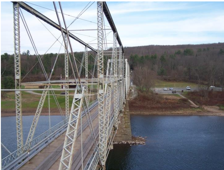
Photo 2 - Skinnners Falls Bridge: Downstream Elevation (Looking East)
