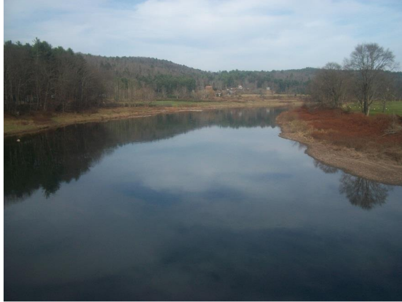
Photo 7 - Skinners Falls Bridge: View of Channel Looking Upstream
