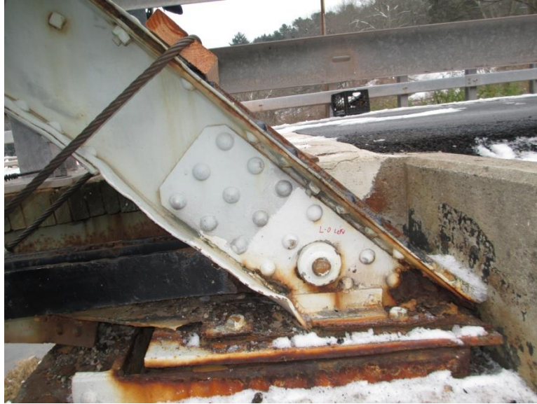
Photo 29 - Skinners Falls Bridge: Near Abutment Left Truss
