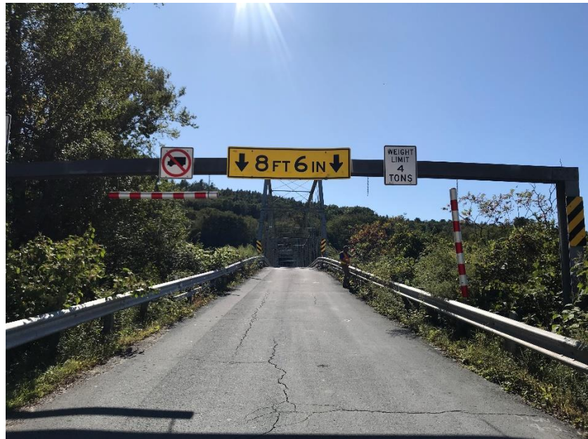
Photo 6 - Skiners Falls Bridge: Headache Bar at NY Approach
