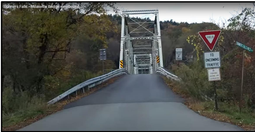
Figure 2: New York Approach geometry with a view west of the approach on the east (New York) side of the bridge.
