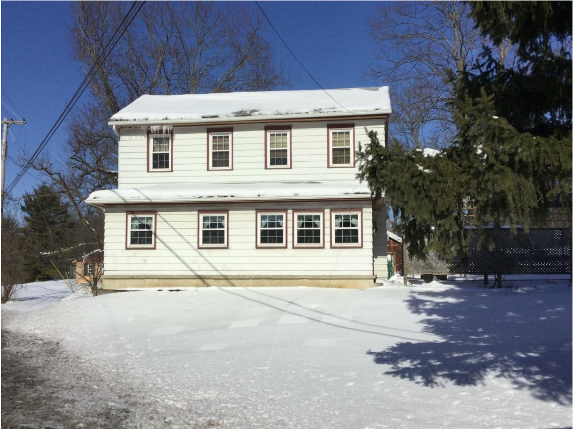
View of the dwelling, looking northwest.
