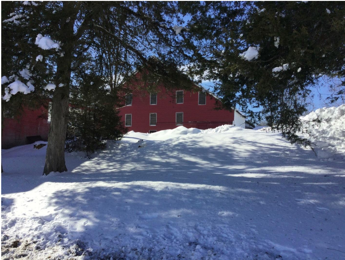
View of the barn at Key No. 059201, looking southwest.
