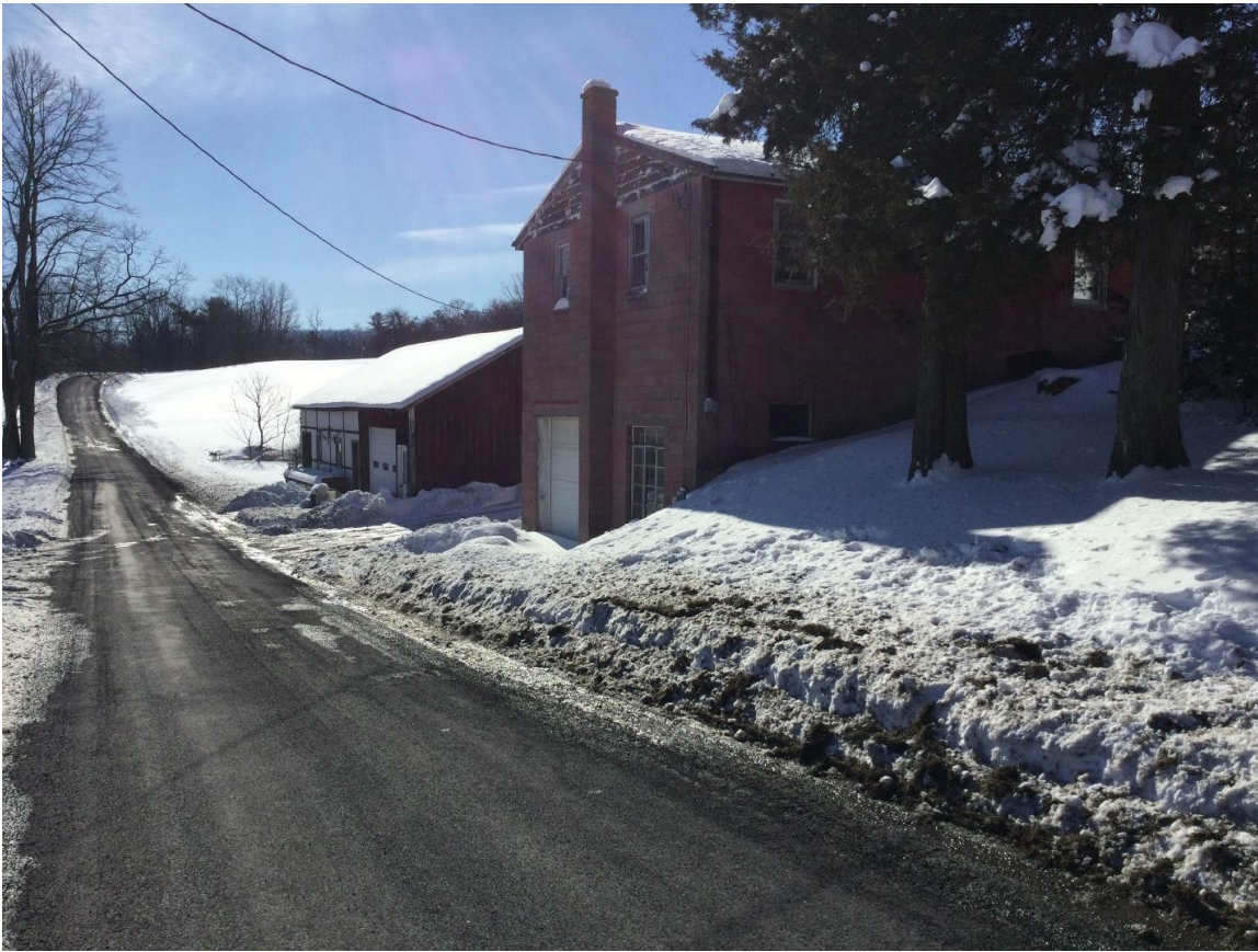
View of the mid-20 th -century outbuildings at Key No. 059201, looking southeast.
