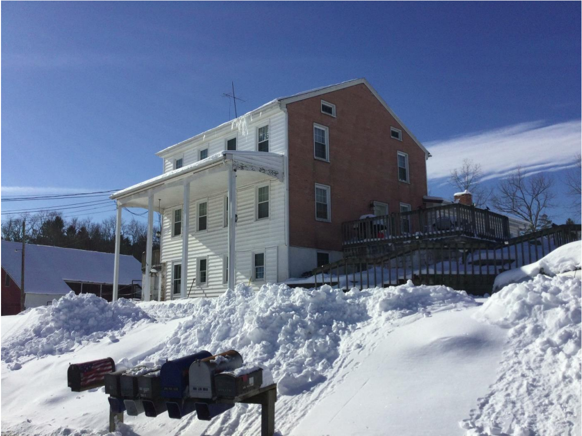
View of the dwelling at Key No. 059201, looking south.
