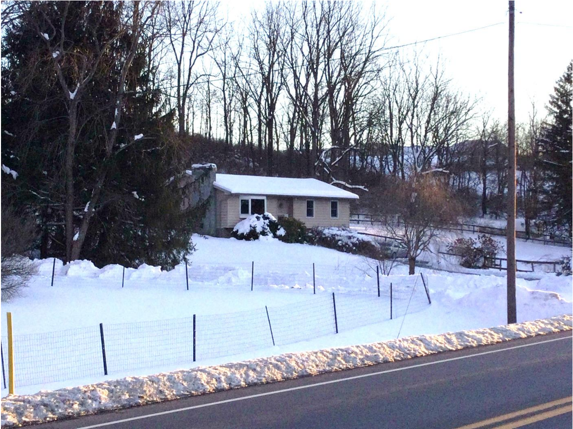
View of the dwelling at Key No. 058395, looking southwest.
