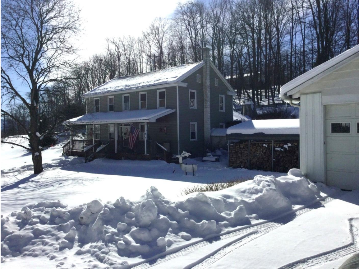
View of Key No. 058305, looking southeast.
