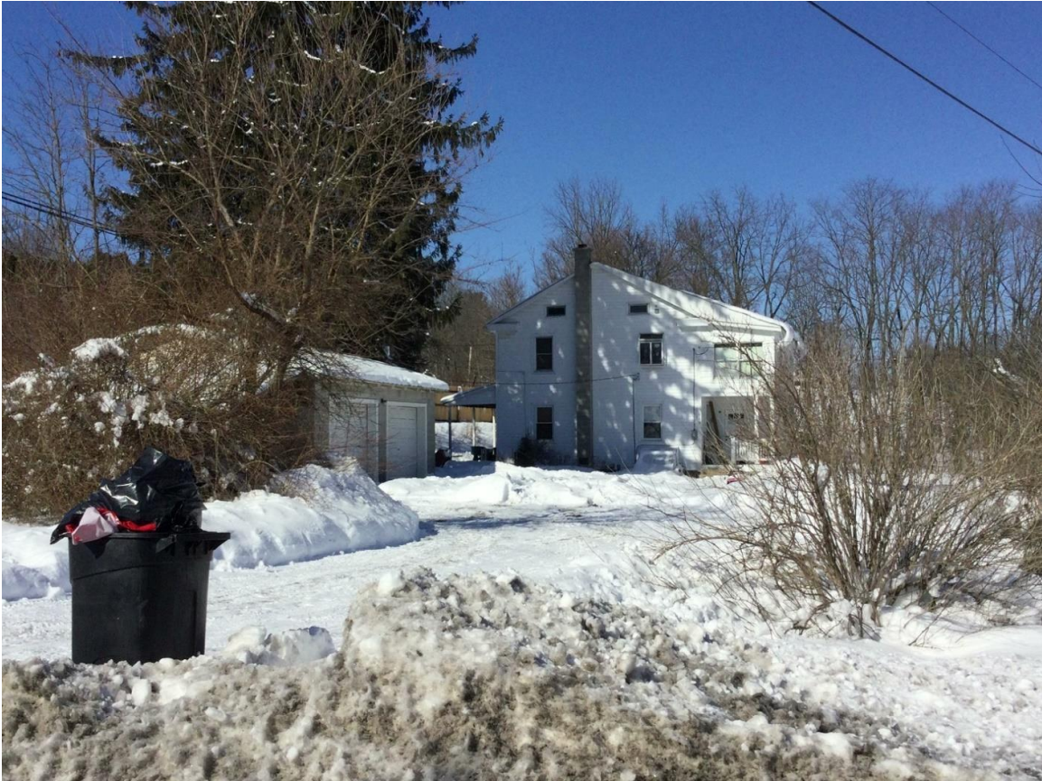
View of the dwelling, looking northwest.
