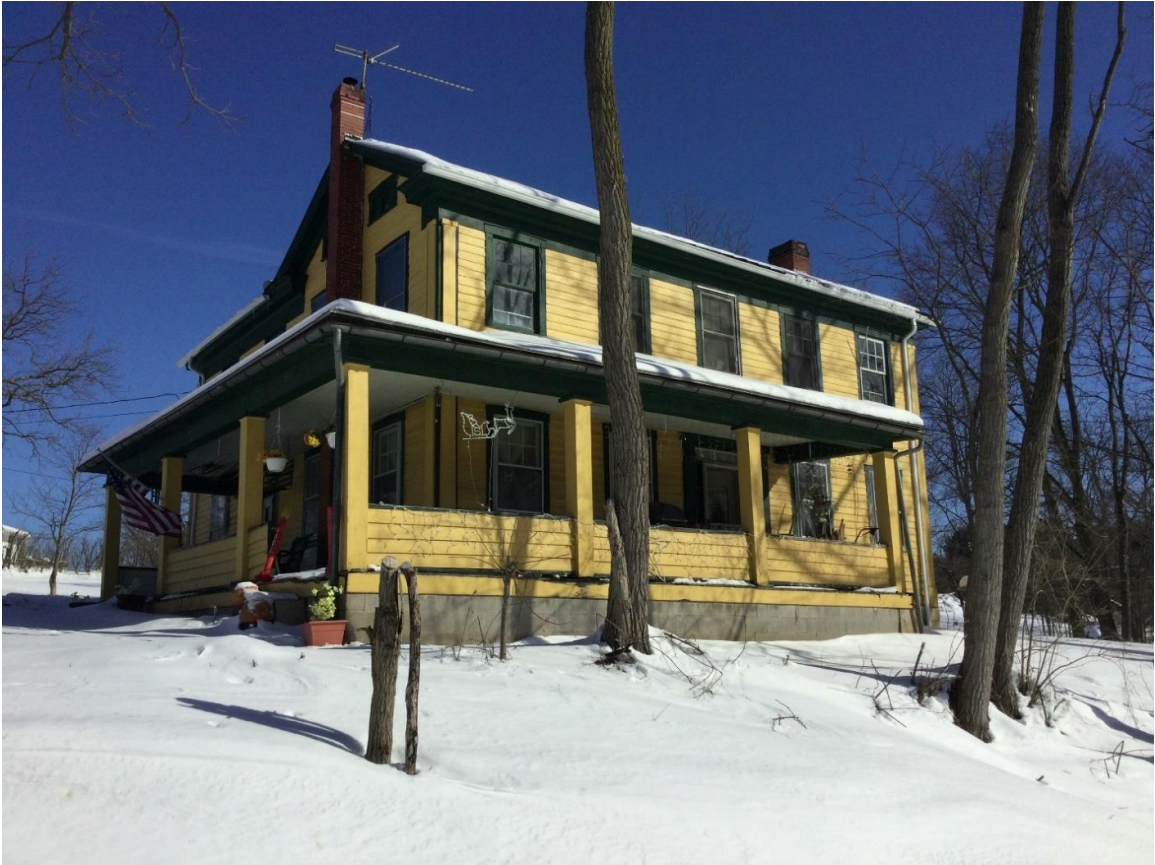
View of Key No. 058306, looking northeast.
