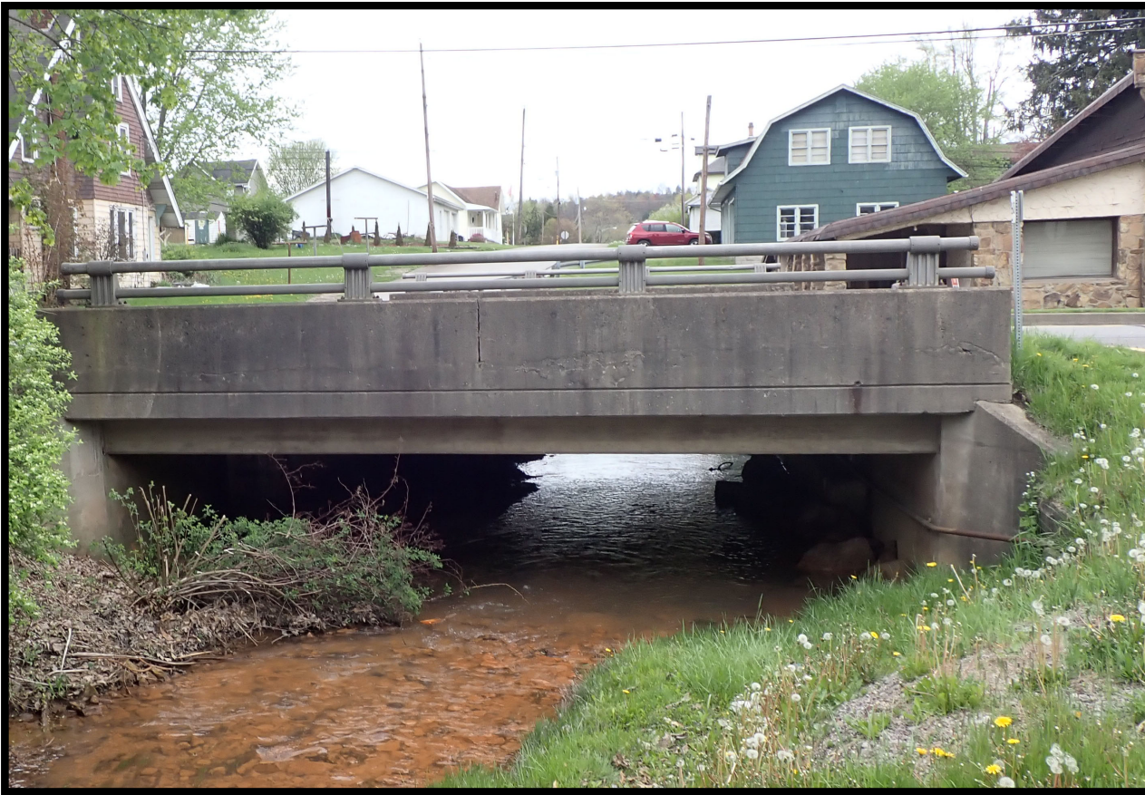
Bridge - Looking West (Downstream)
