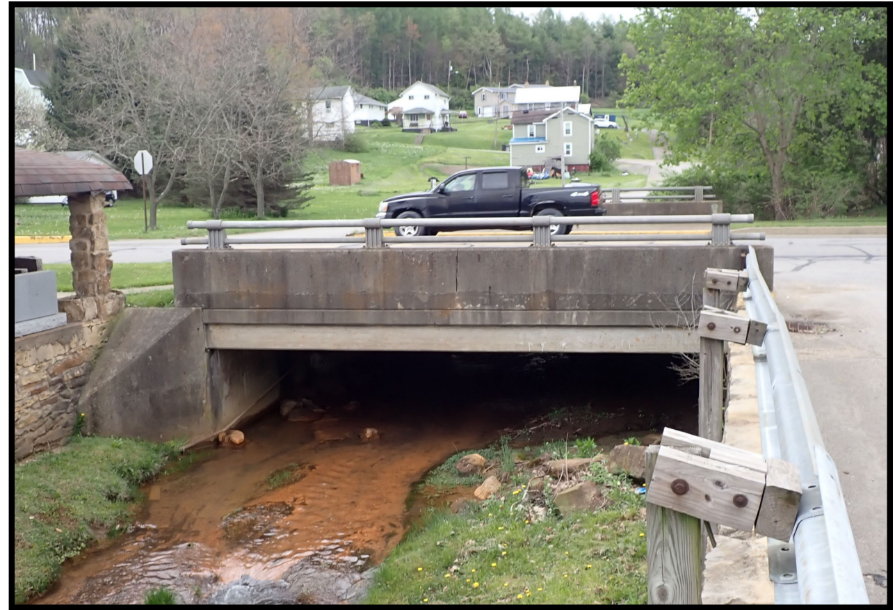
Bridge - Looking East (Upstream)
