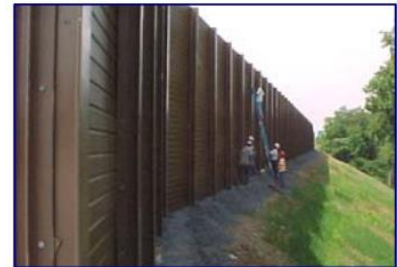
Construction of the Carsonite® sound wall system on I-81
