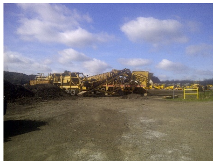
Concrete Crushing Operations
