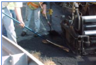
Placement of HMA with 5% Post-Consumer Shingles
