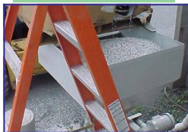
TRPA Material being added to the Hot Mix Asphalt
