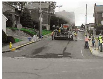
View of the 21 st Street Project during construction
