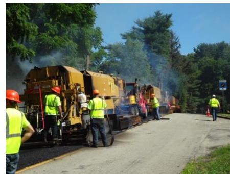
View of HIP Process at the Allegheny County Project Site
