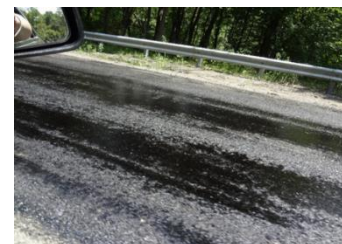
Scarified Asphalt Surface during construction of the Allegheny County Project Site
