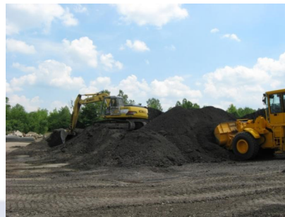
Examples of RAP stockpiling and processing.
