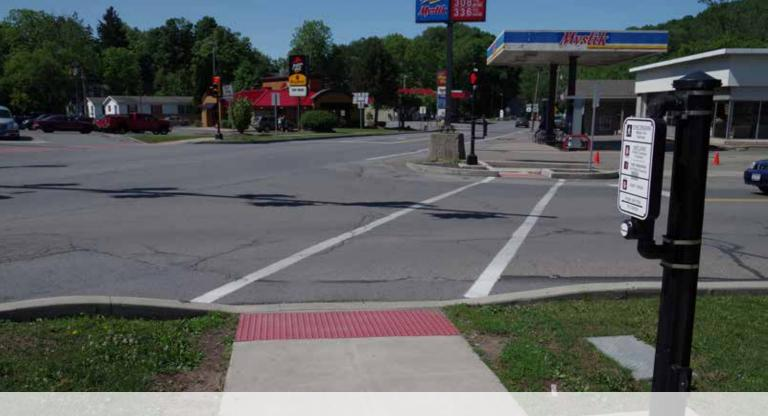
▲ Accessible signal pushbuttons are within reach of a person in a wheelchair—without blocking ramps or sidewalks—and easy to push.
