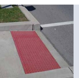
Detectible warning surfaces for vision-impaired pedestrians became an ADA requirement in 2001. In Pennsylvania, one ADA-compliant curb ramp costs \$5,500 on average.
