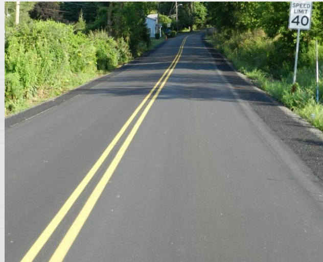
--SR 1029 Bradford County (Before and after upgrade)
