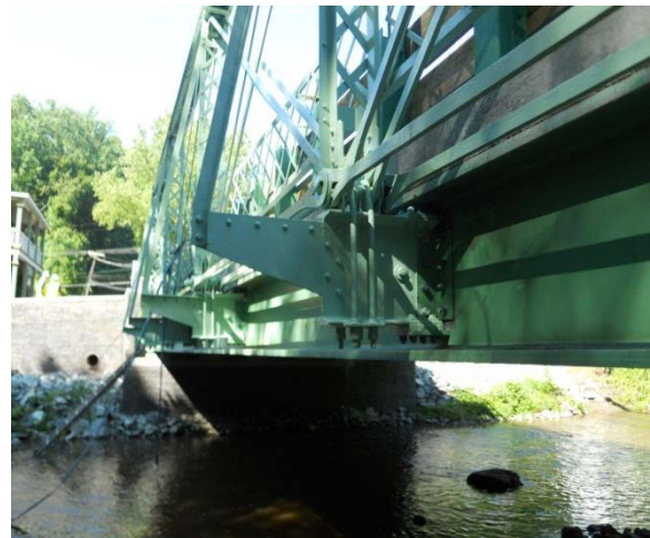
Truss Line Attached to Fascia Stringer.
