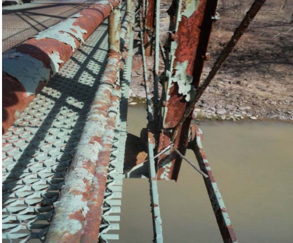
Typical Bottom Chord Connection Detail.
