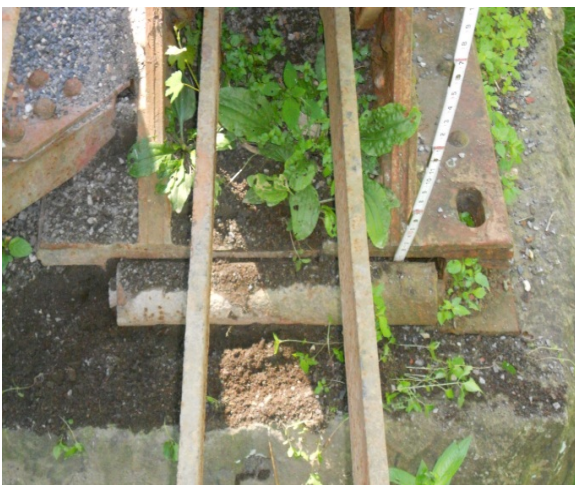
Typical Expansion Bearing.
