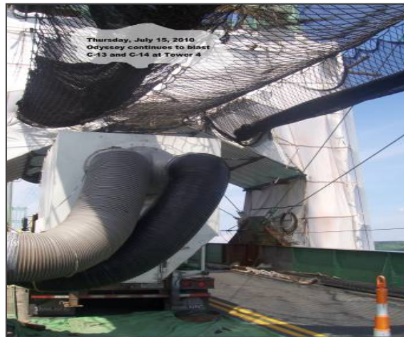
Containment and Vacuum System Required for Lead Based Paint Removal.
