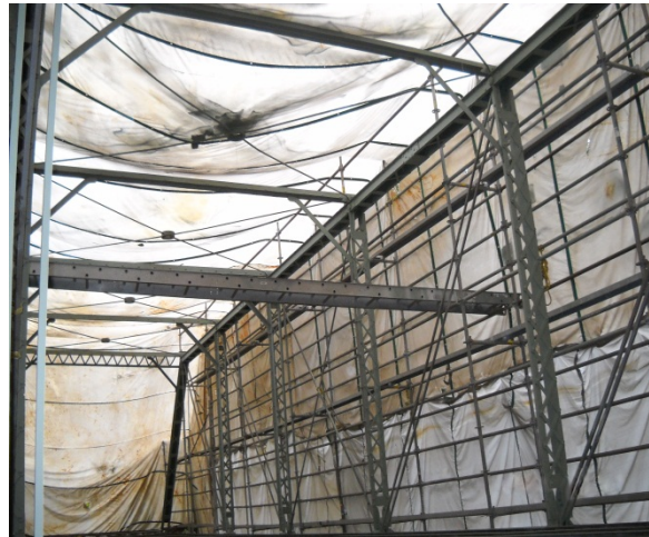
Interior View of Containment System with Scaffolding for Access.
