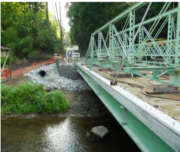
Salvaged Truss Line Ready for Attachment to Fascia Stringer.
