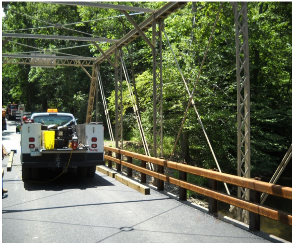
Crashworthy Metal Bridge Railing.
