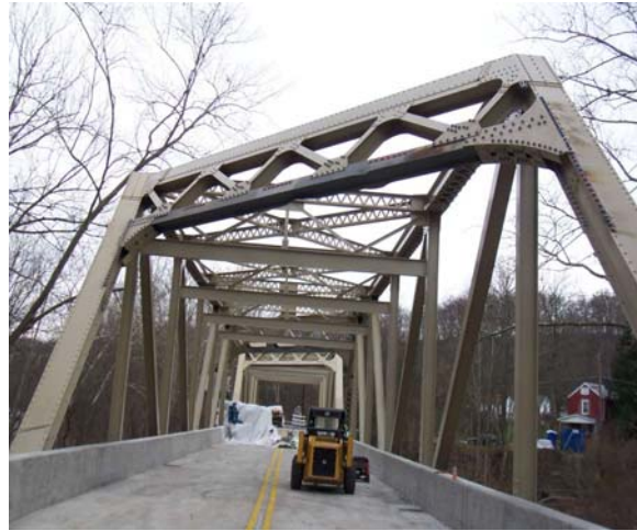
Modified Portal and Sway Bracing System Modified.
