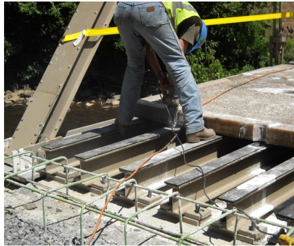
Installation of FRP Deck System.
