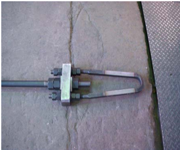
Truss Replacement Member Connection Assembly.
