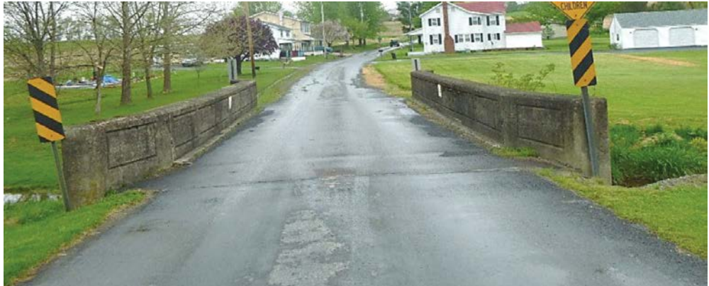
Source: PennDOT Inspection Report
