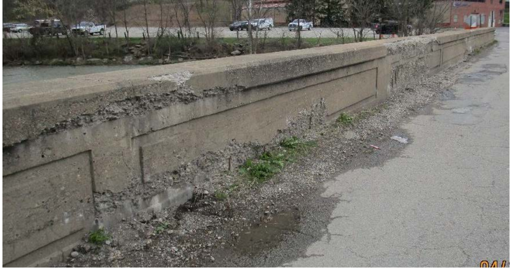
Source: PennDOT Inspection Report
