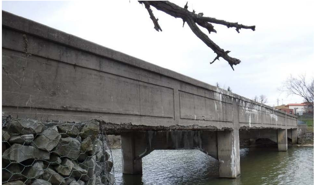
Source: PennDOT Inspection Report
