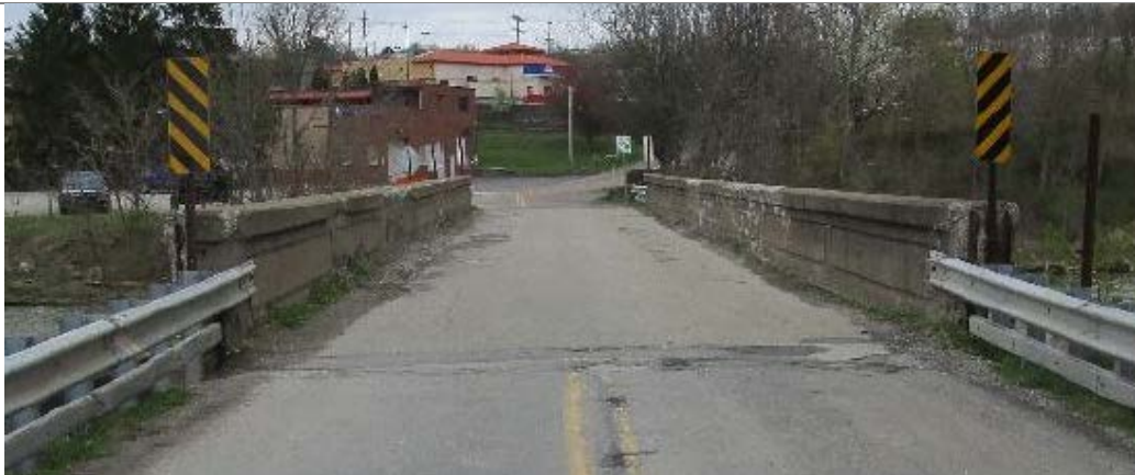
Source: PennDOT Inspection Report
