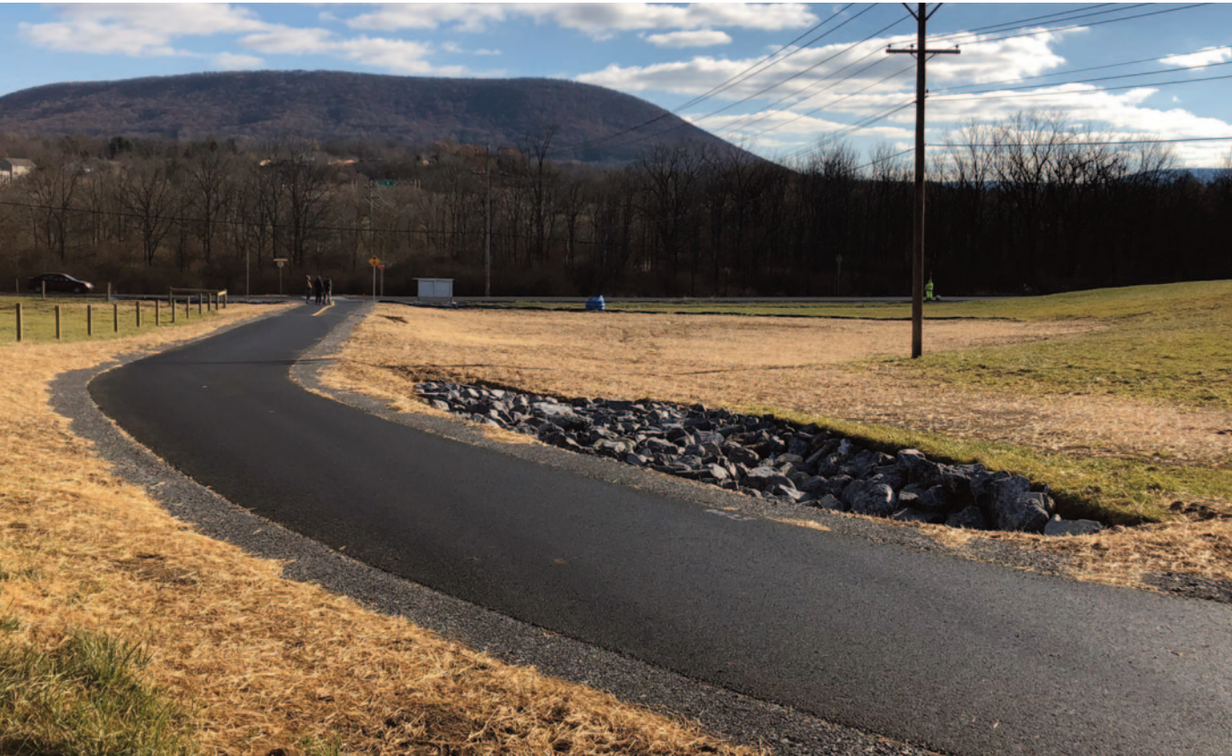
Figure 28: Completed Bike Trail
