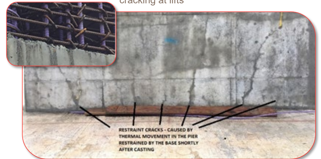
Thermal design to prevent restraint cracking at lifts
