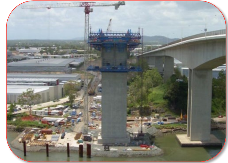
Thermal design to prevent restraint cracking at lifts
