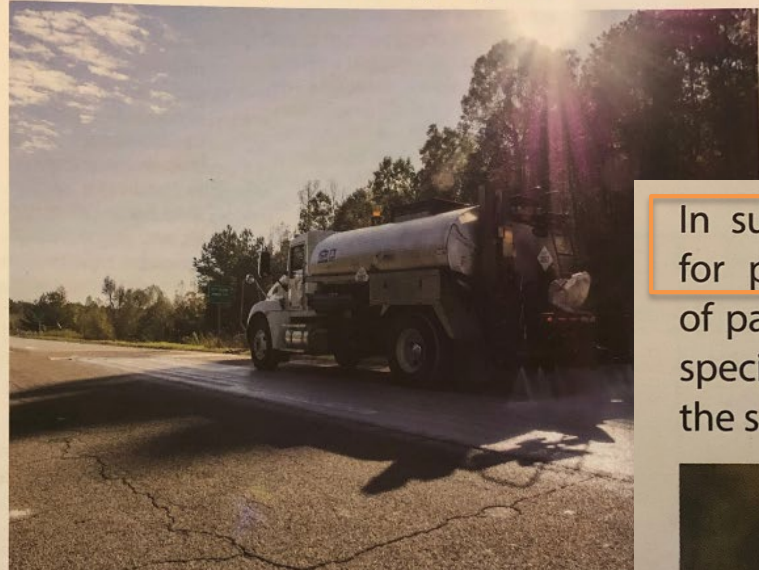
Delta Mist™ rejuvenator is applied to Section S3 of the NCAT Test Track.
