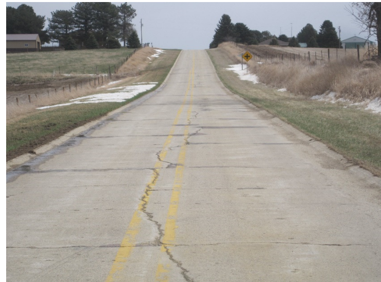
Old US 20, Woodbury County, 2014
