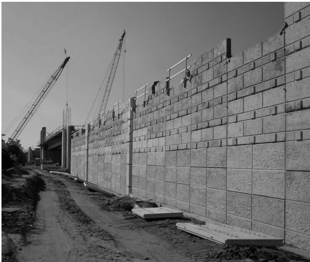
Figure 2-17. MSE wall construction on Mn/DOT Crosstown Project, 2008.
