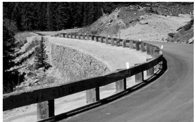
Figure 2-23. Guanella Pass architectural concrete faced wall.
