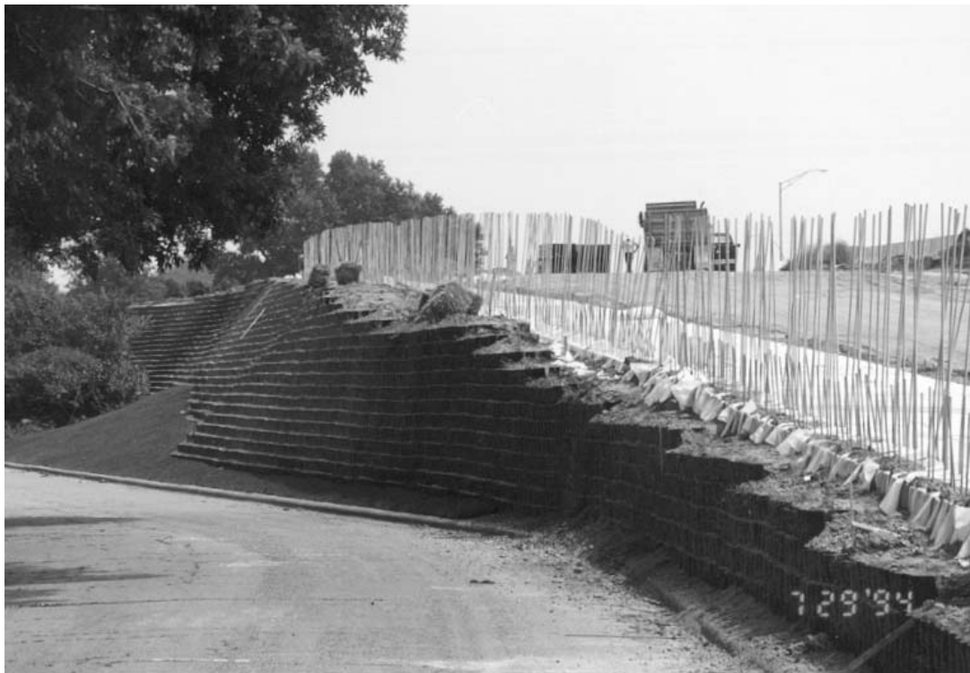
Figure 3-9. Geocell face unit with vegetation.
