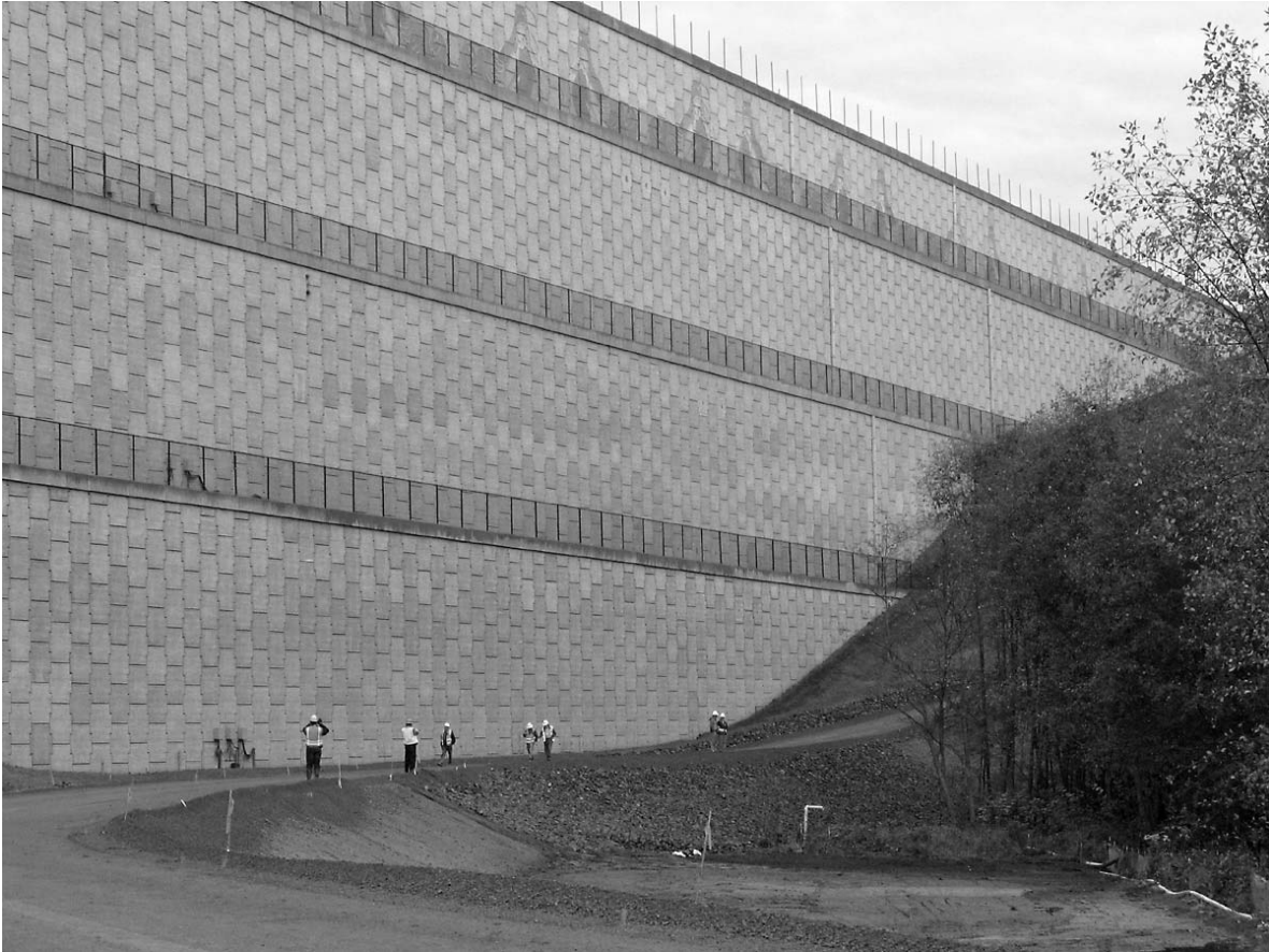
Figure 2-21. SeaTac Airport runway extension MSE wall.
