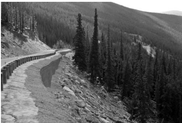
Figure 2-22. Guanella Pass wire-faced wall.
