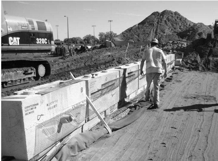
Figure 3-8. Large, wet-cast concrete face unit with embedded reinforcement connectors.
