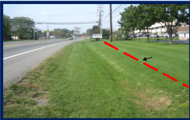
Figure 1.2.1- Storm water conveyed by parallel ditch along road.
