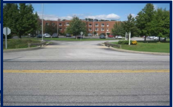
Figure 1.1.2- Culvert conveys water under driveway.
