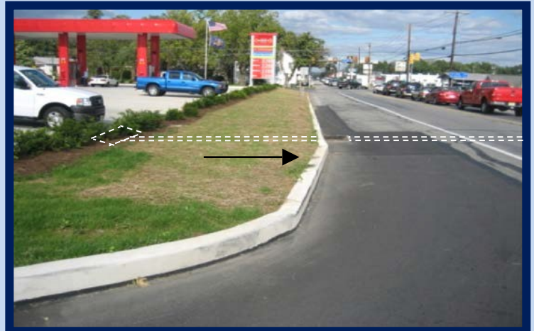
Figure 1.3.2- Site storm water directed into PennDOT Right-of-Way through enclosed surface storm water facilities tied into an existing inlet which is part of a larger storm water system.
