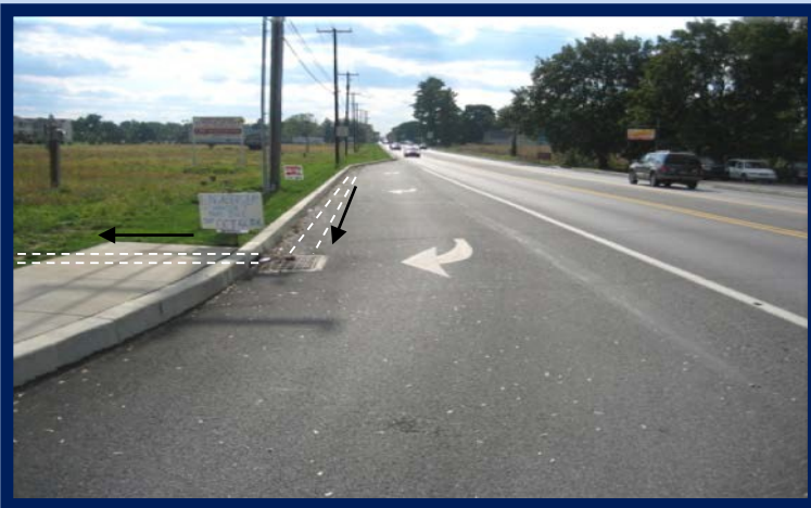
Figure 1.4.1- New enclosed surface storm water installed with curb gutter as part of widening for right turn lane.
