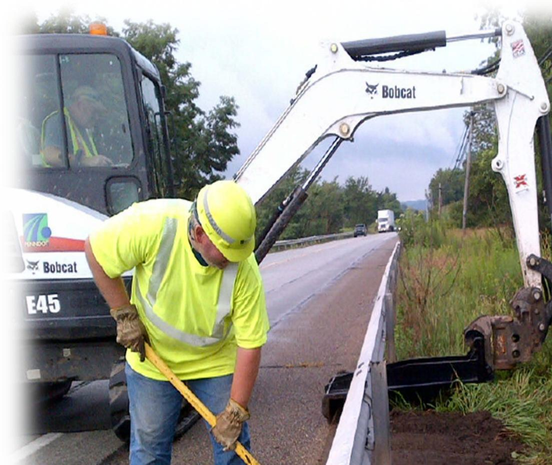
The side dozing attachments were designed for the mini and full-size Excavators to increase production and promote more efficient operations.
