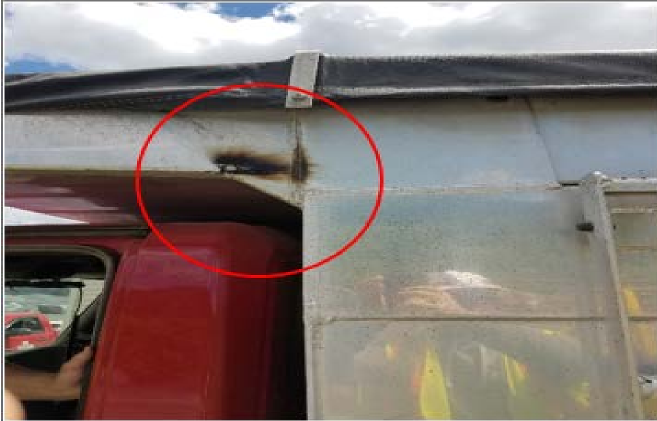
Burnt Marks from Power Wire
