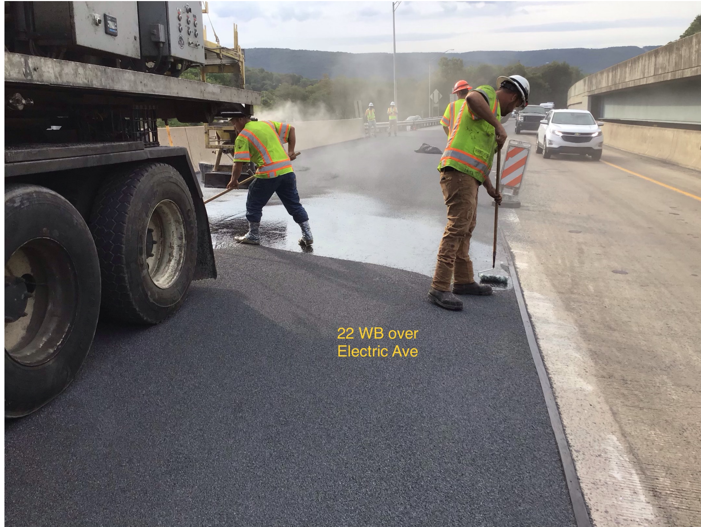
Applying Epoxy Surface Treatment
