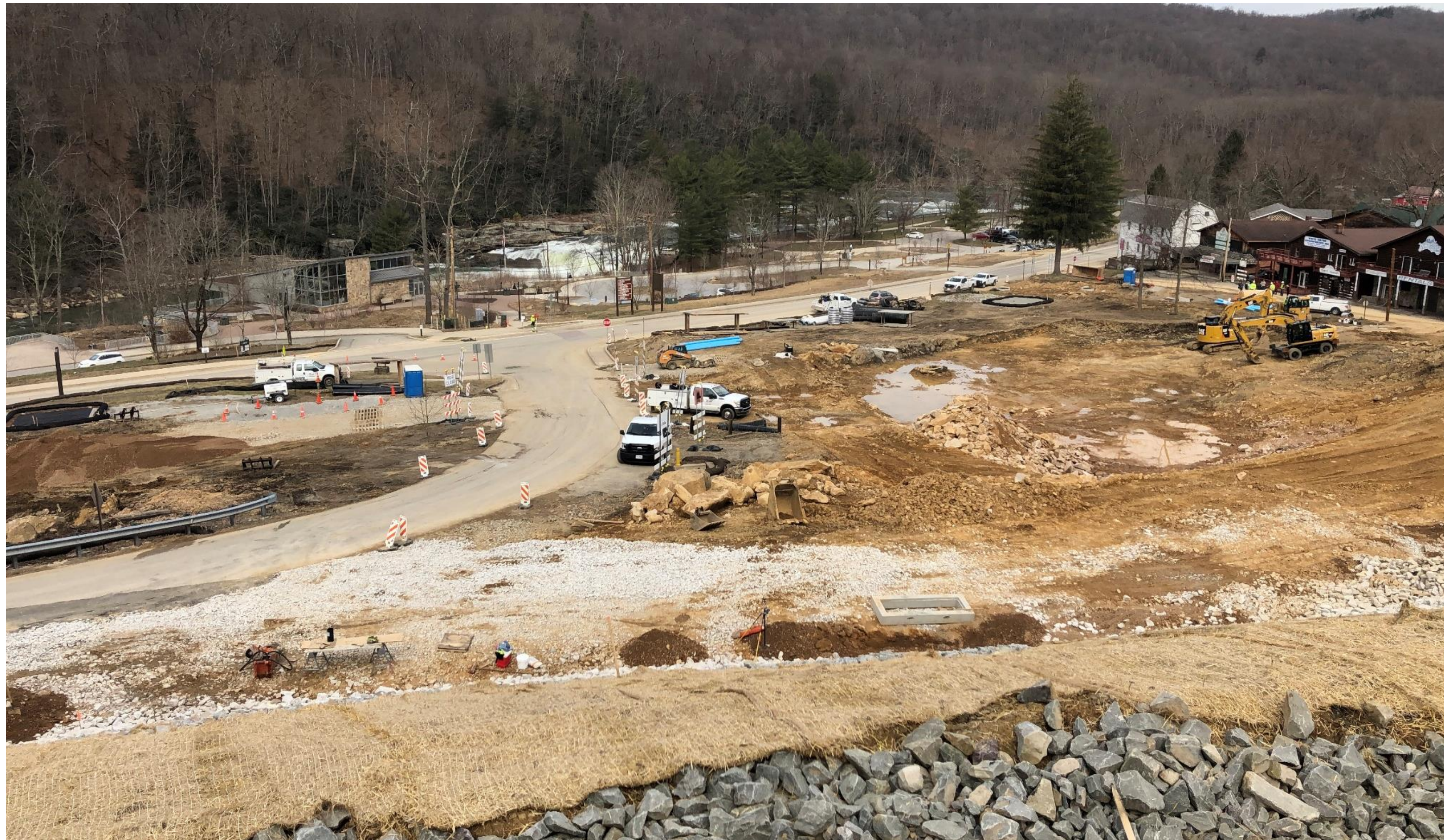
Construction of the Green Infrastructure Parking Lot and Relocated Sugarloaf Road
