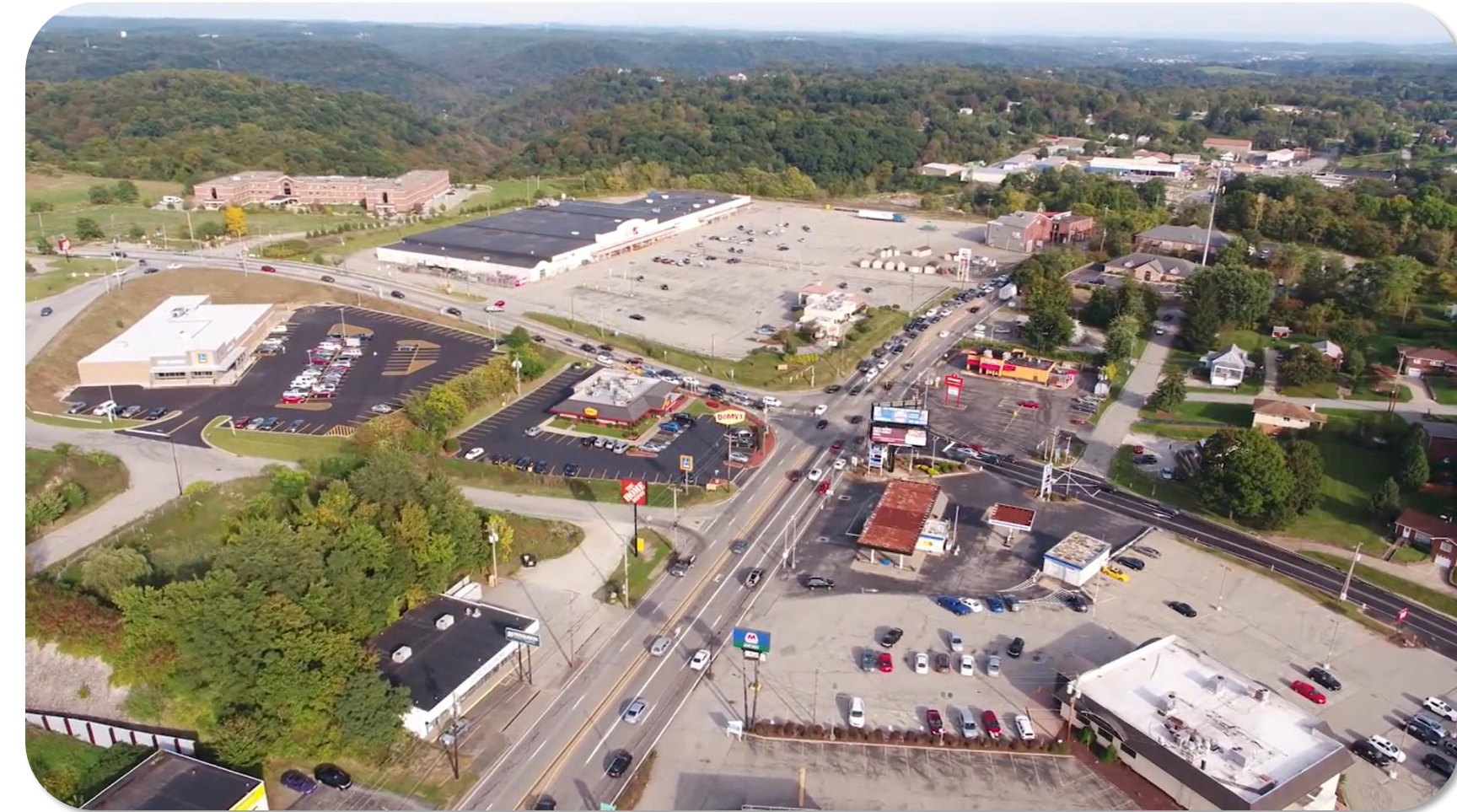
Existing Intersection of US-30 and SR-48, Allegheny County, PA Source: Route 30 Projects Existing Conditions Video
