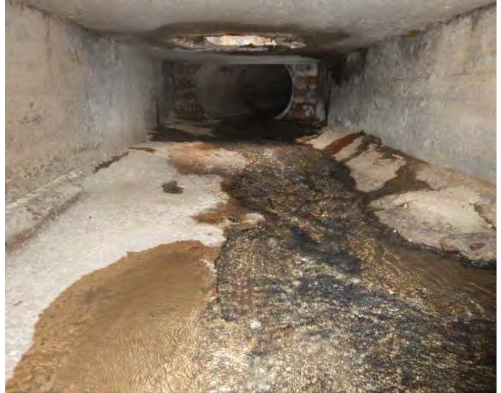
Condition of existing structure with scour – Looking upstream near middle of structure
