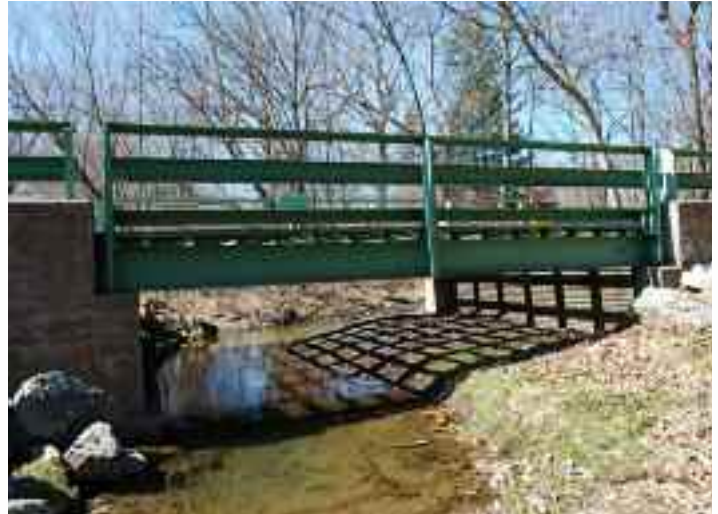
Northampton County will replace 28 bridges and rehabilitate five structures using P3 project delivery.
