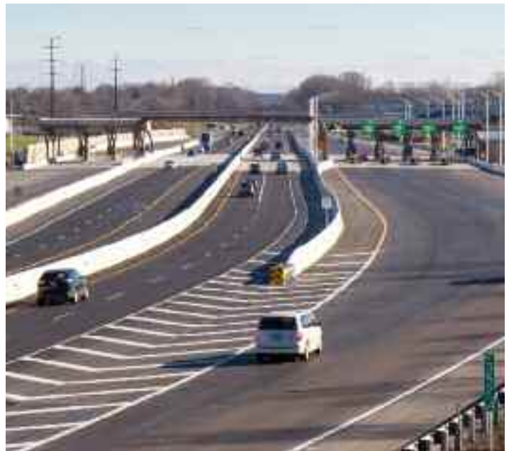
The selected private entity will install fiber optic cable and a wireless network throughout the PTC's 550-mile corridor.
