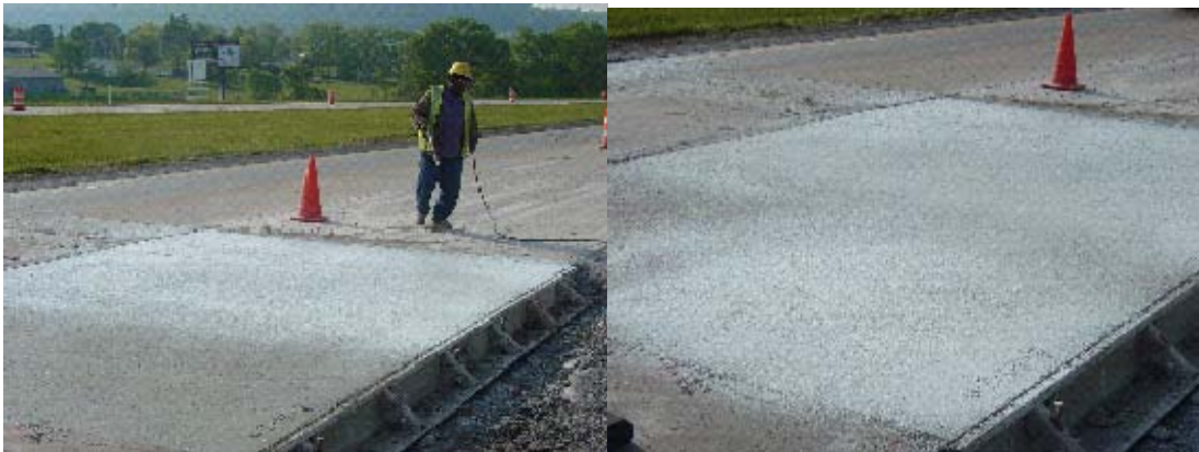
Photographs 20 and 21, The application of the white curing compound after finishing.
