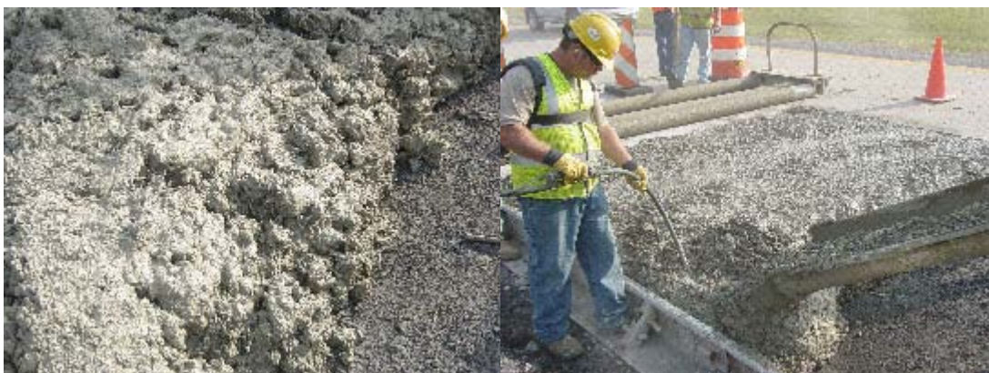
Photographs 16 and 17, The Tuf-Strand fibers in the freshly placed concrete just prior to being consolidated with a concrete vibrator.
