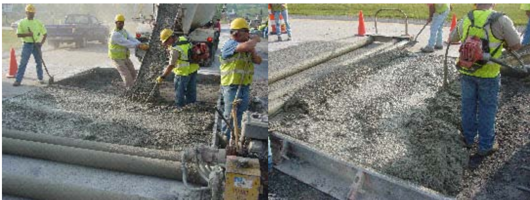
Photographs 14 and 15, The concrete being placed and vibrated to consolidate the plastic concrete in the patch. A power roller screed was used to level the concrete in the patch area.
