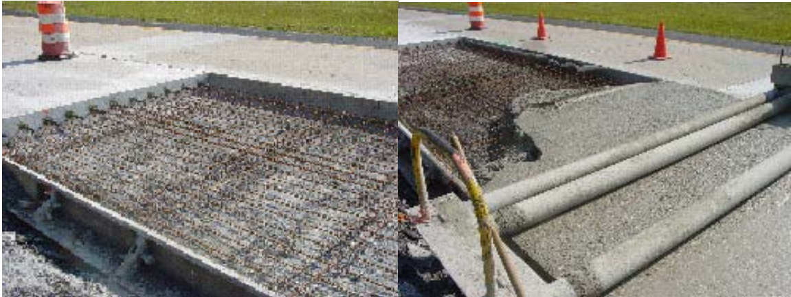
Photographs 1 and 2 illustrate a typically prepared concrete pavement patch area with welded wire fabric reinforcement steel before and during concrete placement.
