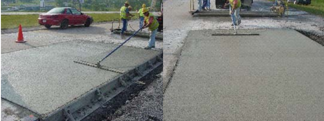
Photographs 18 and 19, The concrete patch being finished with a bull float shortly after the power roller screed was removed.
