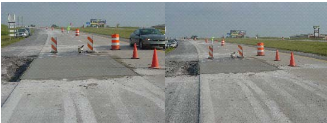
Photographs 22 and 23, The completed concrete patch with the Tuf-Strand fibers.
