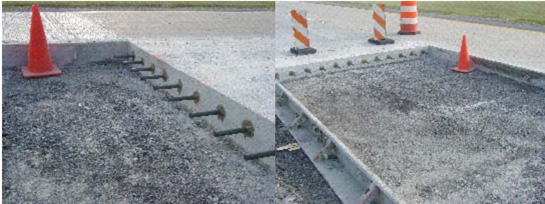
Photographs 12 and 13, The prepared patch area with no welded wire fabric reinforcement steel.
