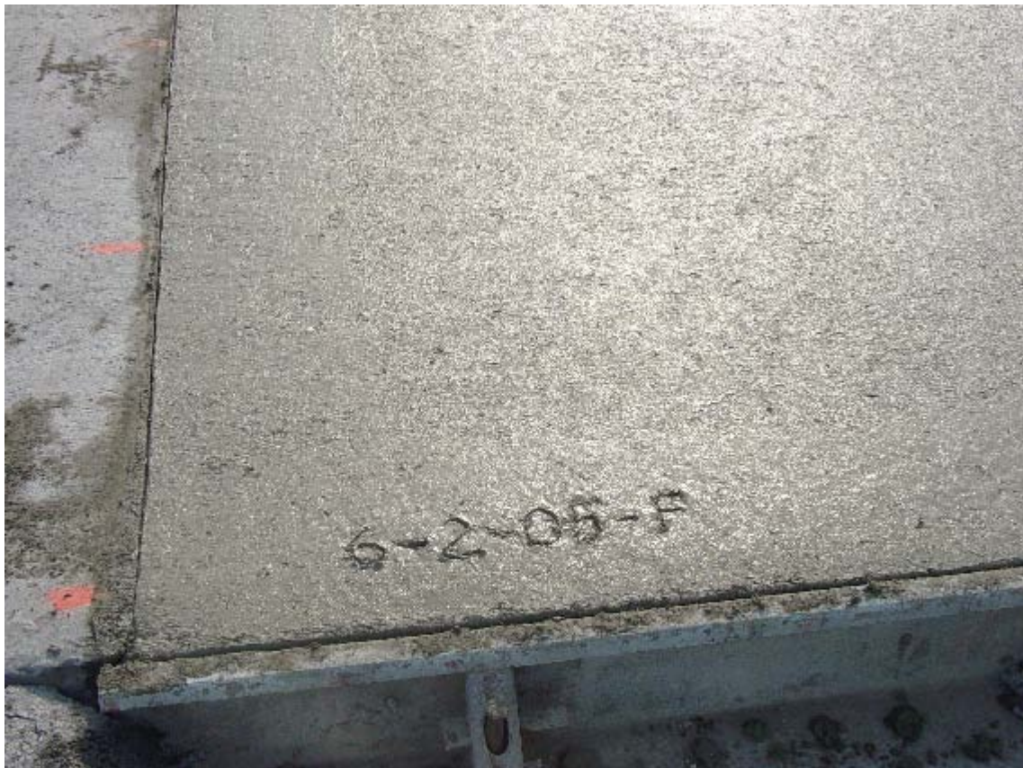
Photograph 11, The patch was inscribed with the date on the corner of the patch to help locate the patch.
