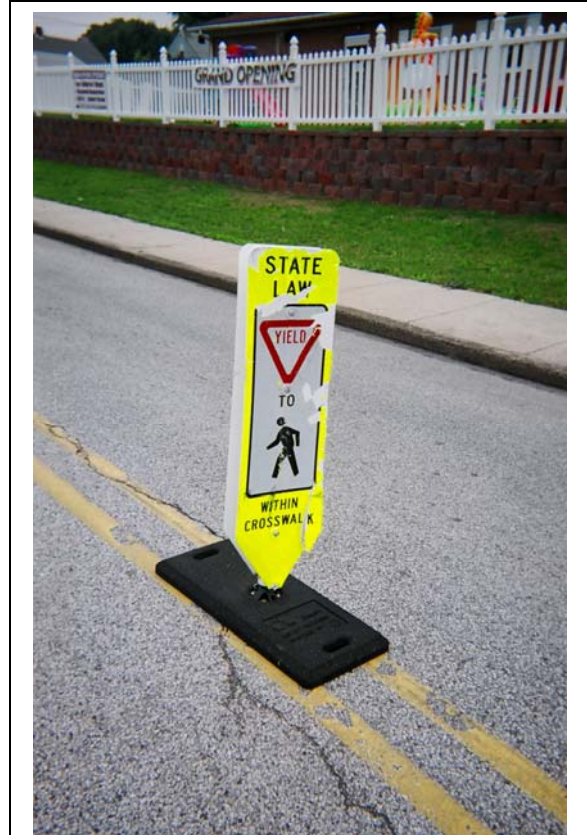
Figure 4-1: Example of YTPCD Damaged by Vehicle
