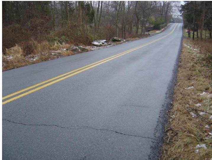
Photo 13, The pavement is exhibiting transverse cracking.
