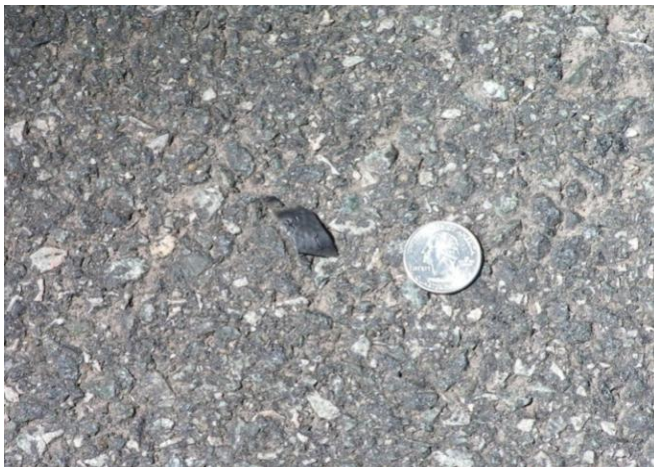
Photo 11, Shredded roofing membrane protruding from the finished roadway.
