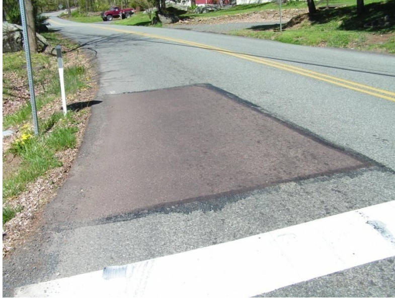
Photo 10, Distressed pavement needed to be patched.
