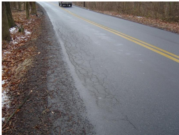
Photo 14, The pavement has additional alligator cracking and rutting.
