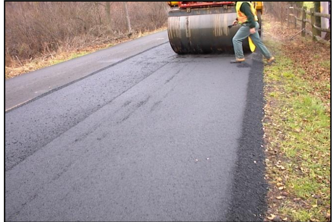
Photo 3, The marred surface of the pavement mat.
