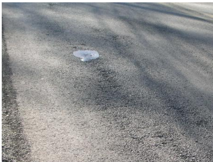
Photo 8, The asphalt road surface of the experimental section appeared to be raveling.
