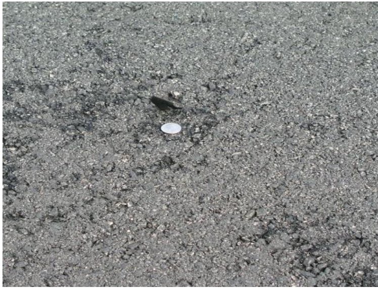
Photo 7, Shredded roofing membrane protruding from the finished roadway.
