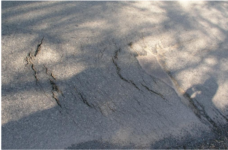
Photo 9, Peeled back asphalt mat at the intersection of Allentown Road and Finland Road.
