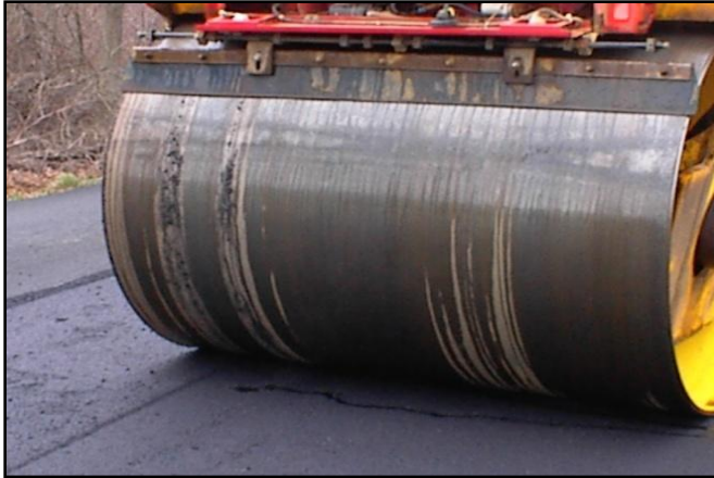
Photo 2, The dry areas on the roller drum picked up the 9.5mm Superpave mix with 5% pulverized shingles material.
