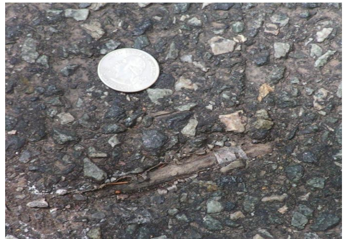
Photo 12, Contaminant in the surface of the pavement.
