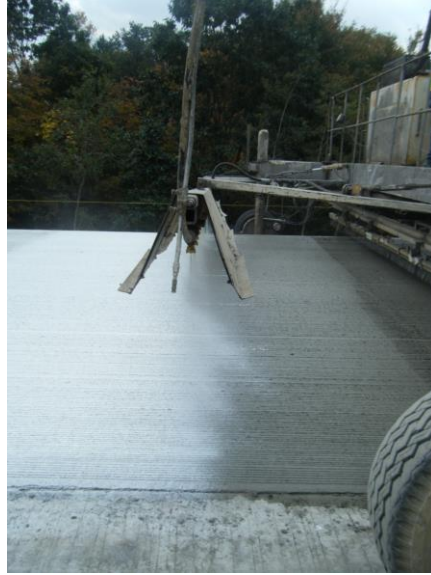
Figure 15. Spray nozzles and wind screen on the cure cart.
