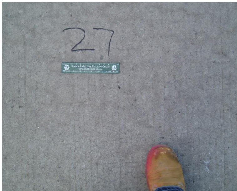
Figure 22. Plastic shrinkage cracking on SR 202 in Chester County, PA.
