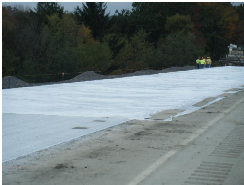
Figure 19. Sheeting used in addition to the curing compound due to impending rain.
