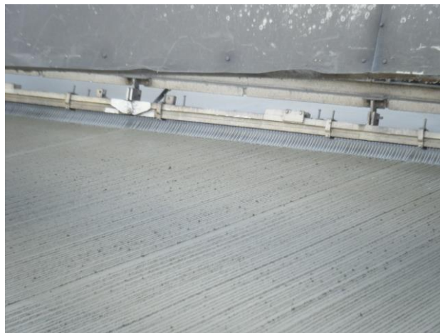
Figure 14. Tining the pavement surface.
