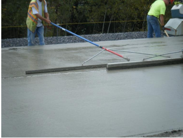
Figure 13. Excess surface water during hand finishing.
