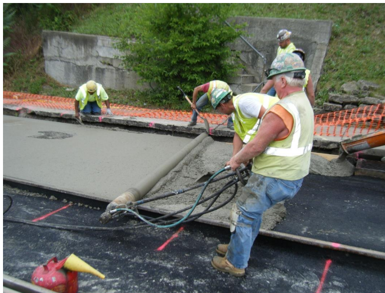
Figure 7. Striking off the concrete and hand finishing.
