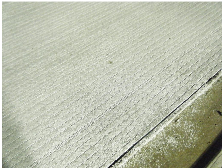
Figure 11. Curing compound on the pavement surface.
