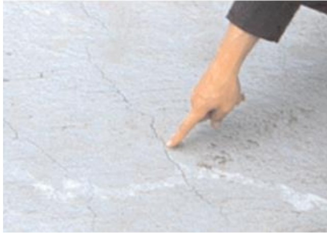
Figure 1. Typical plastic shrinkage cracking (Kostmatka 2002).
