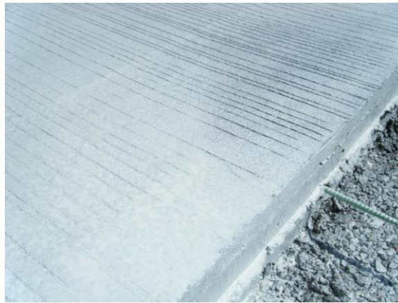
Figure 6. Application of curing compound. Note nonuniform application.
