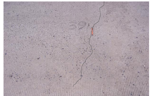
(c) Plastic shrinkage crack number 29 (the crack has been digitally enhanced)
