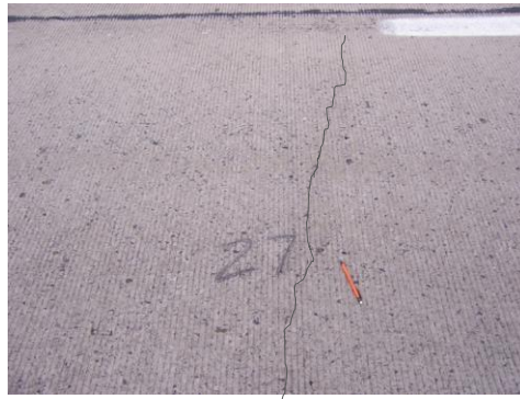
(b) Plastic shrinkage crack number 27 (the crack has been digitally enhanced)
