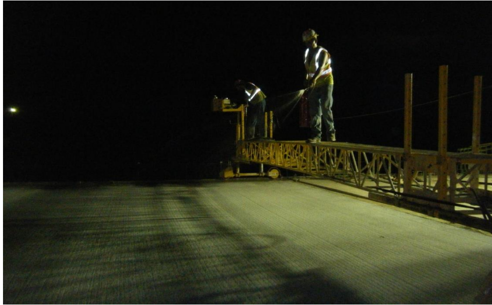
Figure 10. Application of curing compound with hand wand on work bridge.
