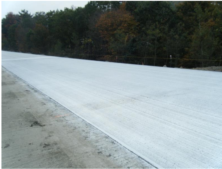
Figure 18. Pavement with applied curing compound.
