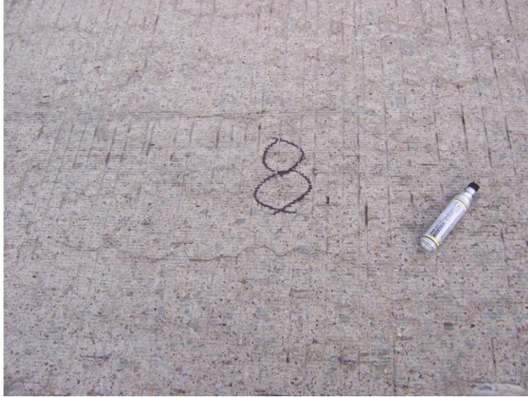
Figure 23. Plastic shrinkage cracking on US 22 in Murrysville, PA.
