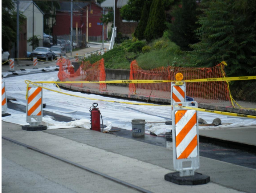
Figure 8. White polyethylene sheet used for curing the roadway section.
