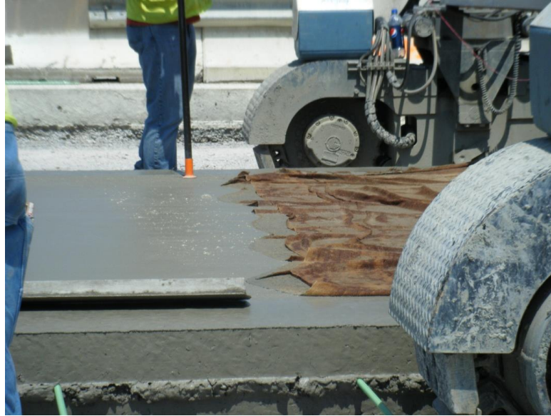
Figure 5. Wet burlap drag for texturing following finishing.
