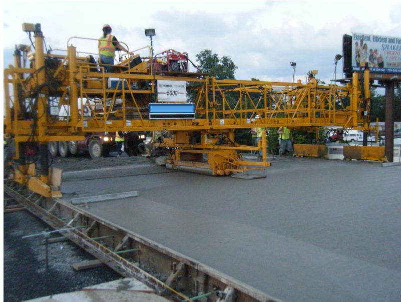
Figure 9. Paving placement equipment.
