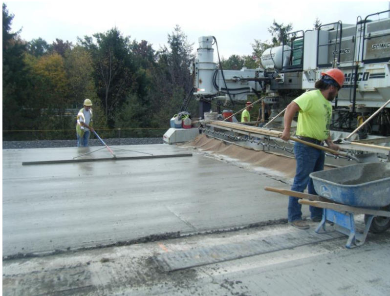
Figure 12. Main paver with burlap drag.
