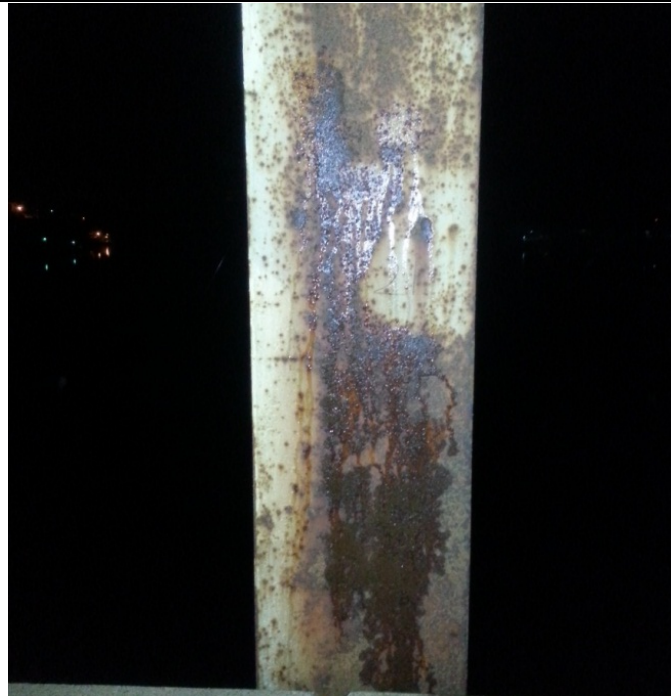
Figure 11: Vanport Bridge, Location 5: Rusted Area Post-wash
