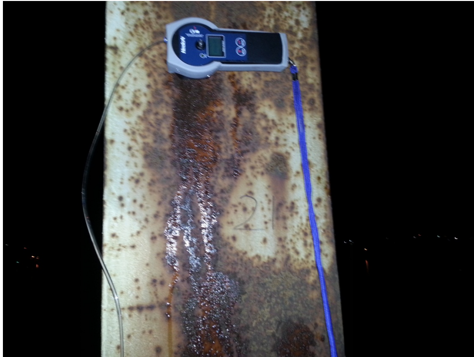
Figure 10: Vanport Bridge, Location 5: Vertical Surface with Significant Corrosion.
