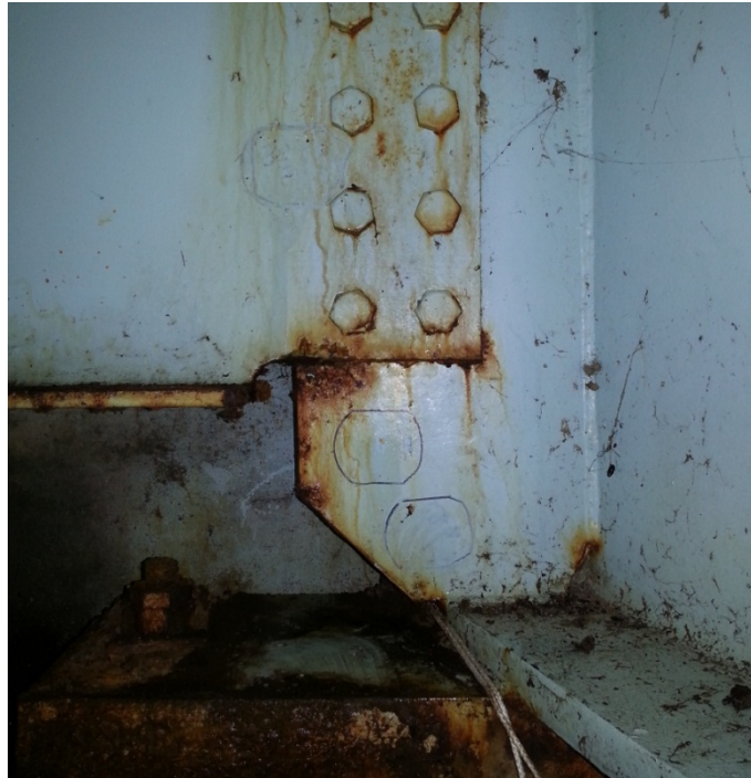
Figure 12 Hassam Road, Location 1, Bearing Stiffener Exhibiting Rust
