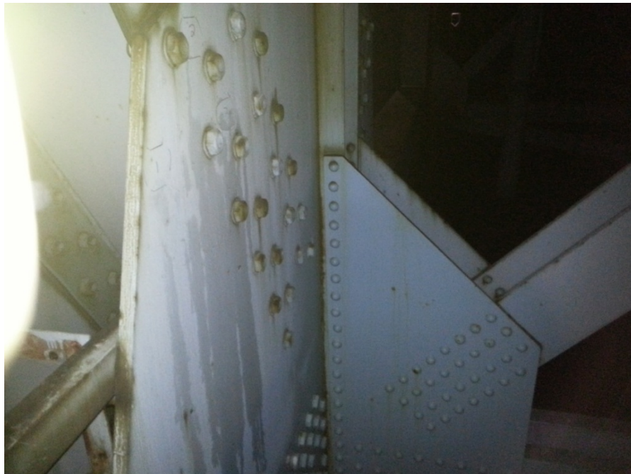
Figure 9: Vanport Bridge, Location 4, Gusset Plate on Inside of Lower Chord
