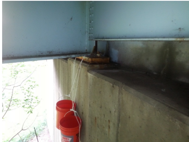
Figure 13: Hassam Road, Location 2: Bearing Stiffener Not Exhibiting Rust
