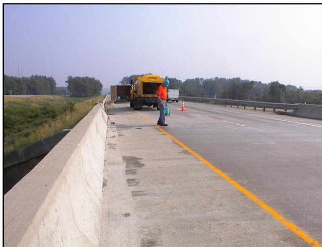
Photo 1, DensiCrete Application on SR 79 Northbound
