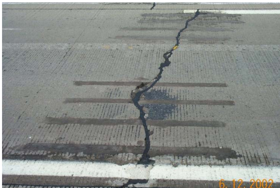
Figure 6: DBR with Minor Spalling and Pop-out
