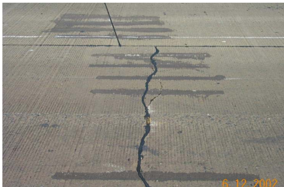
Figure 7: DBR with New Crack
