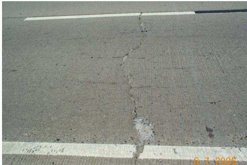
Figure 5.1 Mid-slab Crack at 2240/0107
