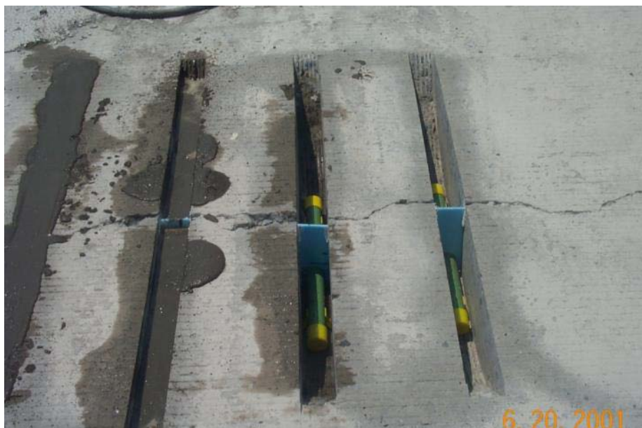
Figure 2: DBR Installation
