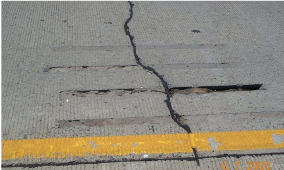
Figure 2.0 Compromised DBR at 2240/0438
