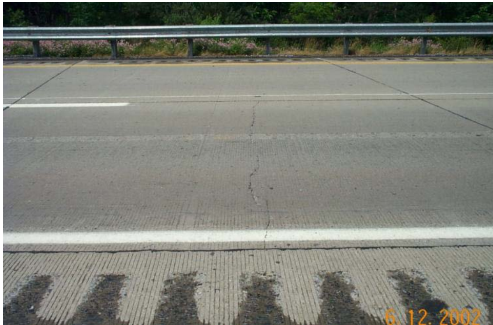
Figure 1: New Crack
