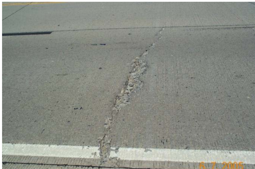
Figure 5.0 Mid-slab Crack at 2240/0070
