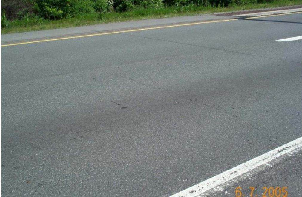
Figure 11.0 Zone 7 - Transverse Cracking at 2244/1791
