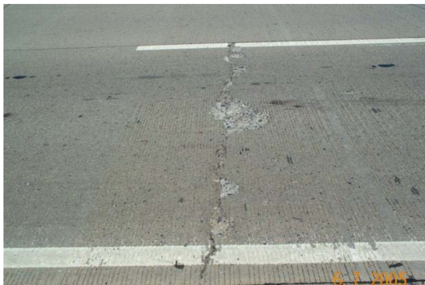
Figure 5.2 Mid-slab Crack at 2240/0168
