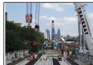
Installation of new guideway on SEPTA's Market Street Elevated Line
